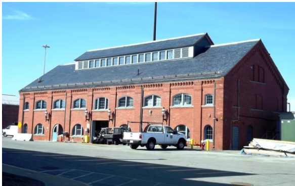
Photo: Field's Point Maintenance Building
