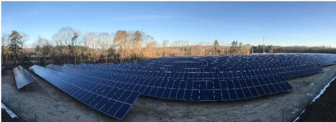
Photo: NBC's Solar Project in Richmond, RI
