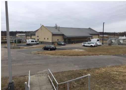
Photo: Current Operations Building
