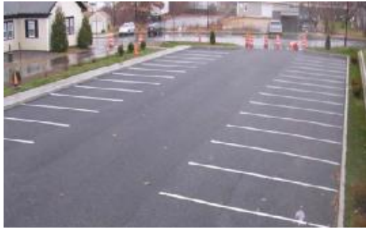
Photo: Permeable Pavement in parking lot
