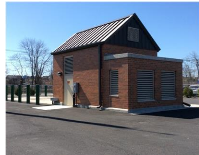
Photo: WCS01 Gate & Screening Structure
