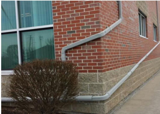
Photo: Downspouts at NBC's Corporate Office Building
