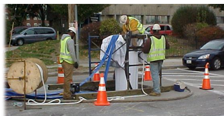
Photo: Infrastructure Repairs
