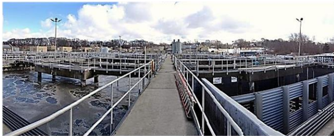
Photo: Aeration Tanks at the Field's Point Wastewater Treatment Facility
