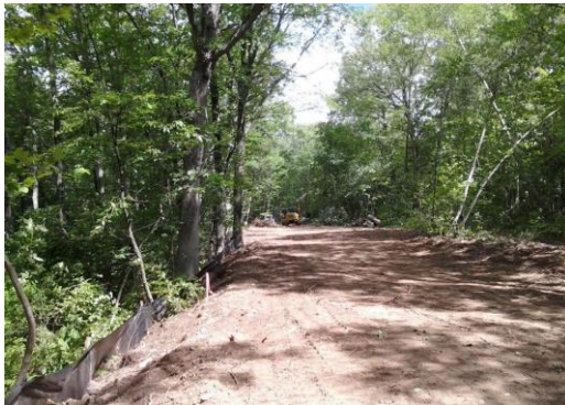
Photo: Easement clearing
