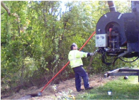
Photo: Interceptor grit removal
