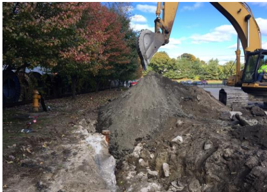
Photo: Construction on the Moshassuck Valley Interceptor
