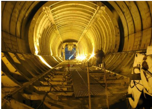
Photo: Phase I Tunnel in Providence
