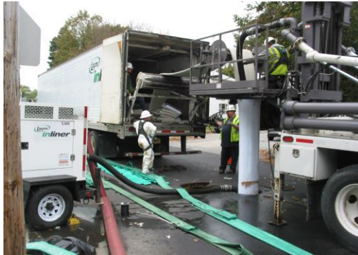
Photo: Rehabilitation of interceptors
