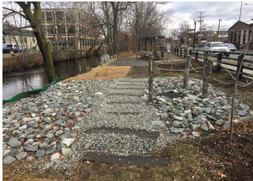
Photo: Surcharge area at Kinsley Ave Providence, RI
