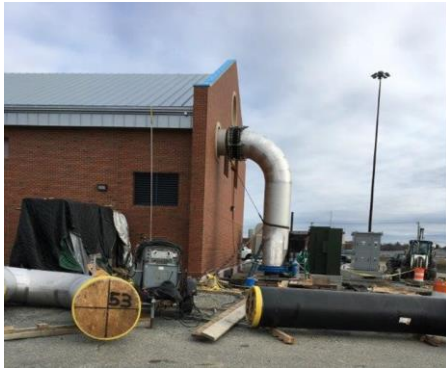
Photo: Blower Building under construction
