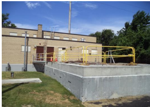
Photo: Omega Pump Station
