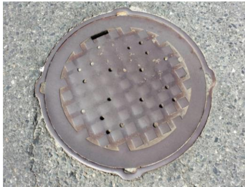
Photo: Municipal Sewer Manhole Cover
