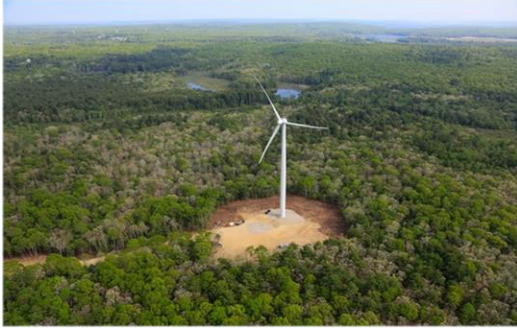
Photo: NBC's "WED 4" turbine in Coventry, RI
