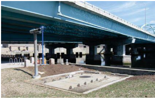
Photo: Siphon Outlet Chamber
