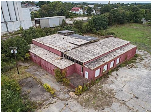
Photo: Existing Structure
