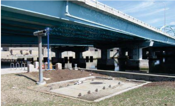
Photo: Siphon Outlet Chamber
