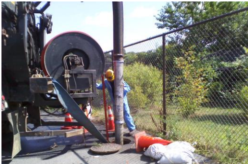
Photo: Interceptor grit removal
