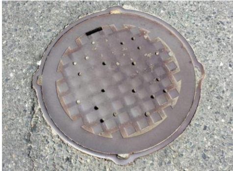
Photo: Municipal Sewer Manhole Cover
