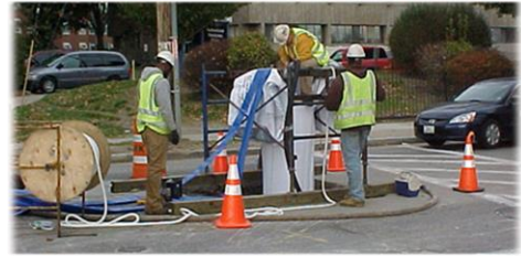
Photo: Infrastructure Repairs
