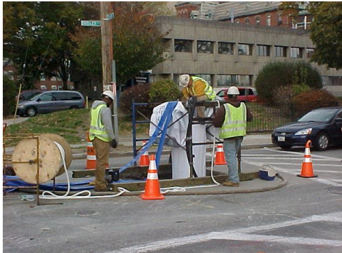
Photo: Conducting Sewer System Repairs
