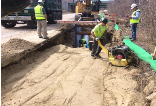
Photo: Construction on Greenville Avenue
