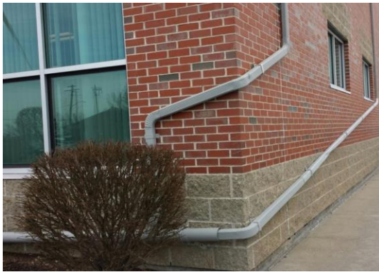
Photo: Downspouts at NBC's Corporate Office Building
