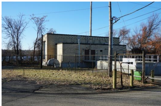
Photo: Omega Pump Station
