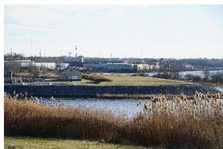
Photo: Bucklin Point WWTF
