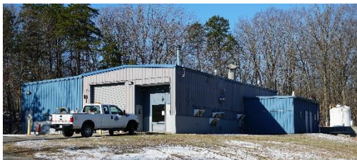
Lincoln Septage Station
