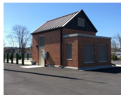
Photo: WCS01 Gate & Screening Structure
