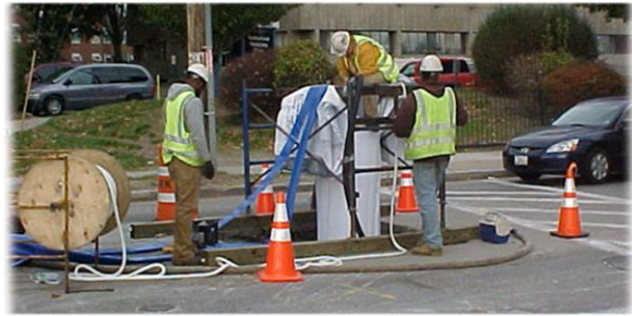
Photo: Collection System Infrastructure Repair
