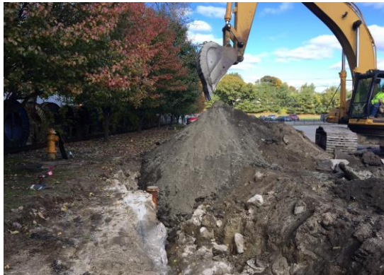
Photo: Construction on the Moshassuck Valley Interceptor
