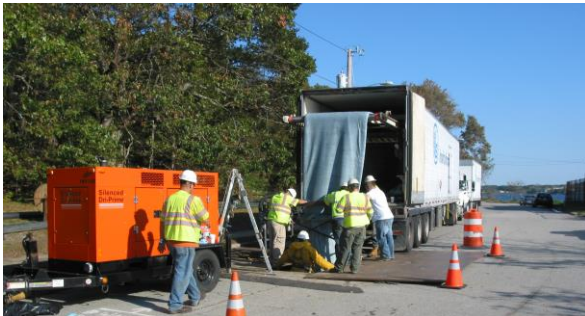
Photo: Rehabilitation of Interceptors
