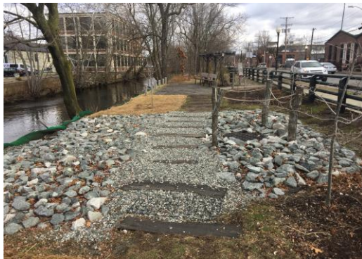
Photo: Surcharge area at Kinsley Ave, Providence
