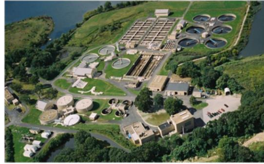
Photo: Bucklin Point Wastewater Treatment Facility
