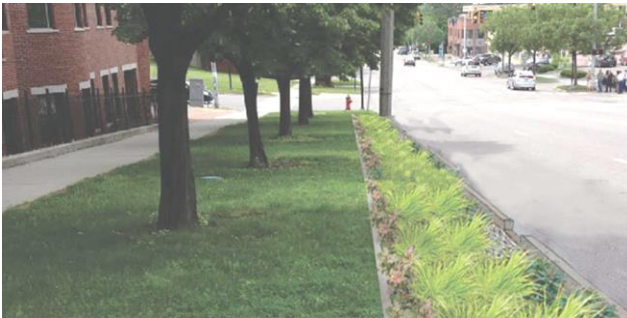
Photo: Example of Green Stormwater Infrastructure
