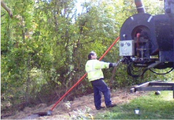
Photo: Interceptor grit removal
