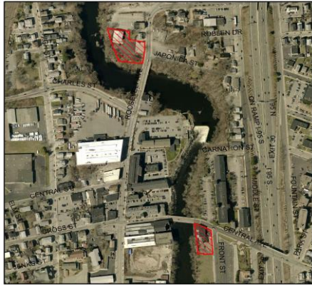
Photo: Demolition Sites
