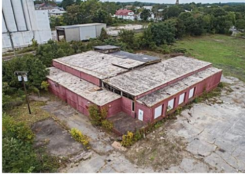
Photo: Existing Structure
