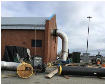
Photo: Blower Building under construction
