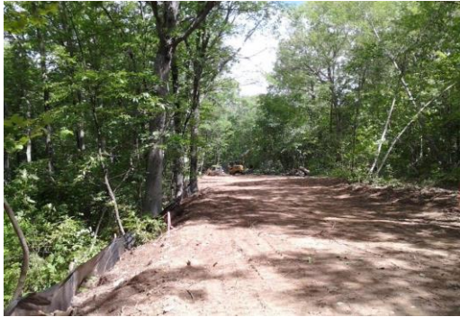
Photo: Easement clearing
