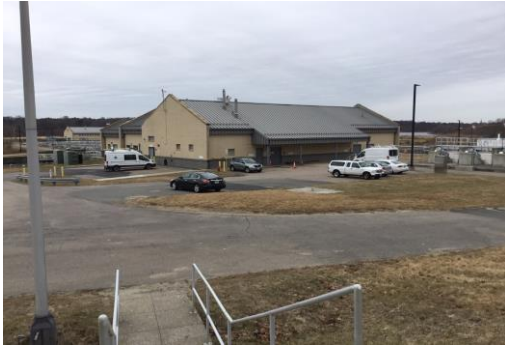
Photo: Current Operations Building
