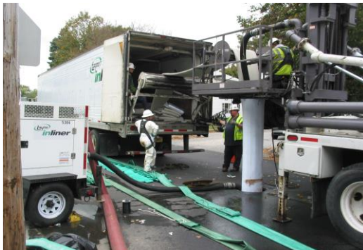
Photo: Rehabilitation of interceptors
