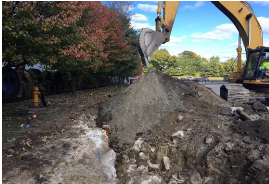
Photo: Construction on the Moshassuck Valley Interceptor
