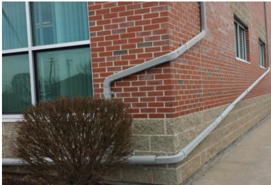
Photo: Downspouts at NBC's Corporate Office Building
