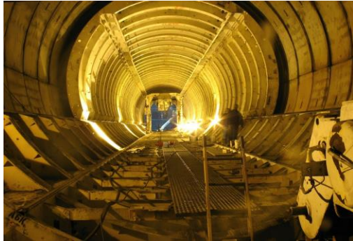
Photo: Phase I Tunnel in Providence
