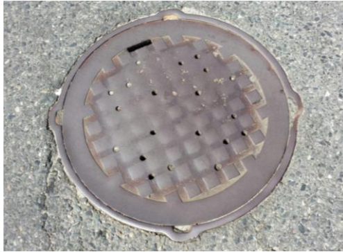
Photo: Municipal Sewer Manhole Cover
