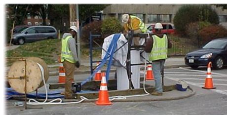
Photo: Infrastructure Repairs
