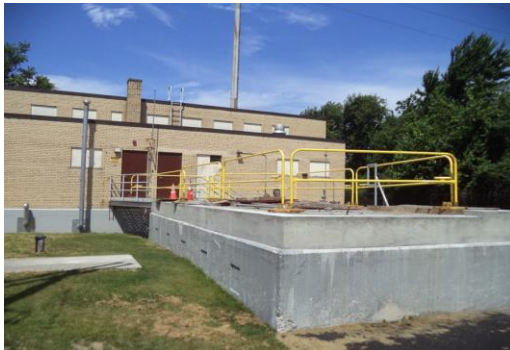
Photo: Omega Pump Station
