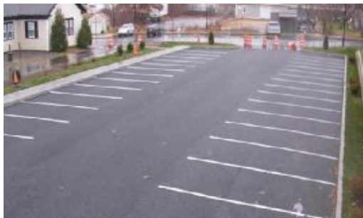
Photo: Permeable Pavement in parking lot
