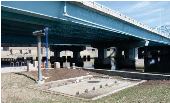
Photo: Siphon Outlet Chamber
