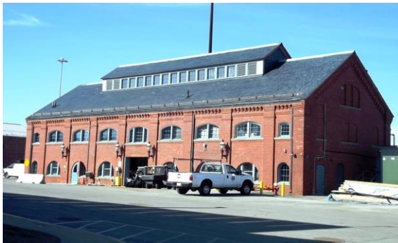
Photo: Field's Point Maintenance Building
