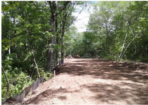
Photo: Easement clearing
