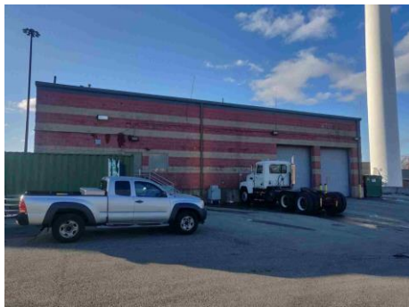
Photo: Sludge Dewatering & Handling Facility
