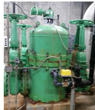
Photo: Water Automatic Strainer
