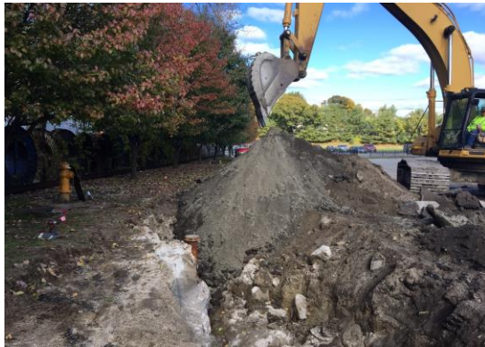
Photo: Construction on the Moshassuck Valley Interceptor
