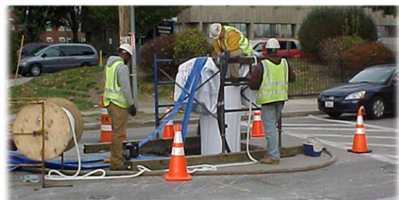
Photo: Collection System Infrastructure Repair
