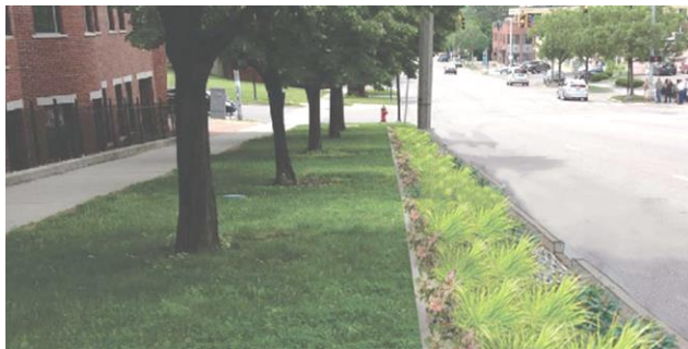
Photo: Example of Green Stormwater Infrastructure
