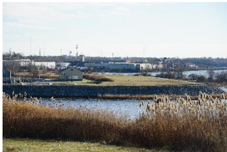
Photo: Bucklin Point WWTF
