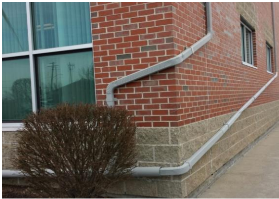
Photo: Downspouts at NBC's Corporate Office Building
