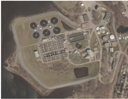
Photo: Existing Clarifiers at Bucklin Point
