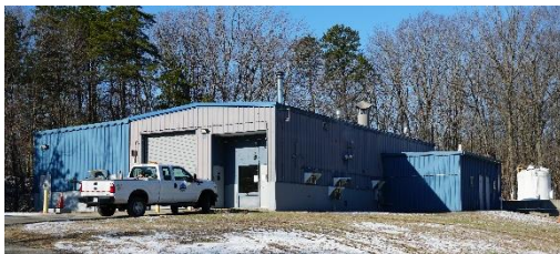
Lincoln Septage Station
