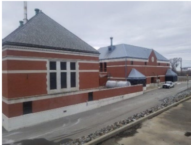
FPWWTF Ernest Street Pump Station
