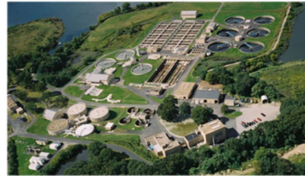
Photo: Bucklin Point Wastewater Treatment Facility
