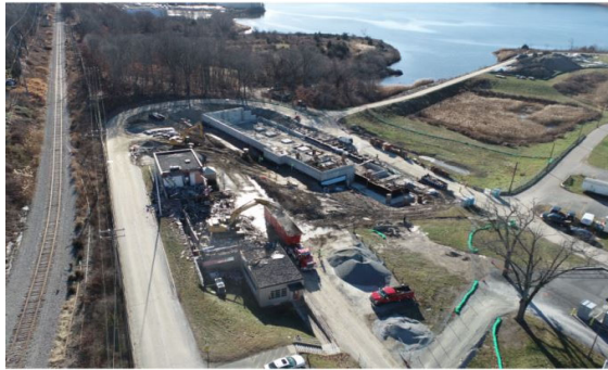
Photo: Operations & Maintenance Building
