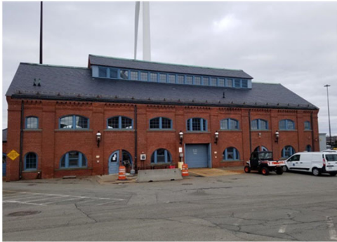
Photo: Existing FPWWTF Maintenance Building
