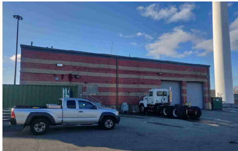
Photo: Sludge Dewatering & Handling Facility
