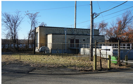
Photo: Omega Pump Station
