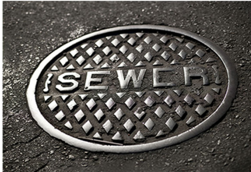
Photo: Municipal Sewer Manhole Cover
