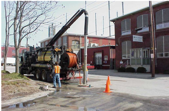
Photo: Interceptor Grit Removal
