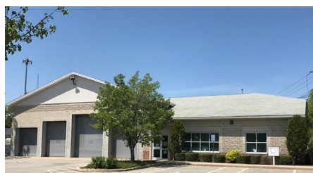
Interceptor Maintenance Building
