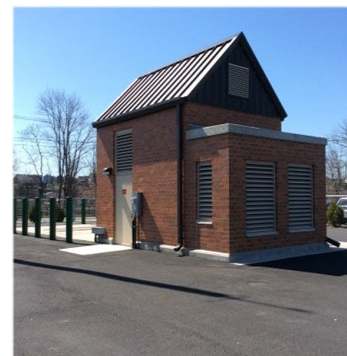
Photo: WCS01 Gate & Screening Structure
