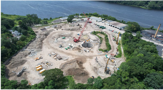
Photo: Pawtucket Tunnel Site
