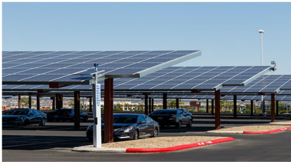
Photo: Solar Carport
