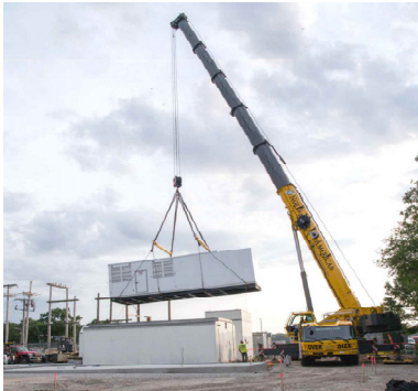
Photo: 2,000 kWh Generator Installation
