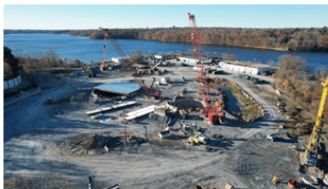
Pawtucket Tunnel Pump Station Site
