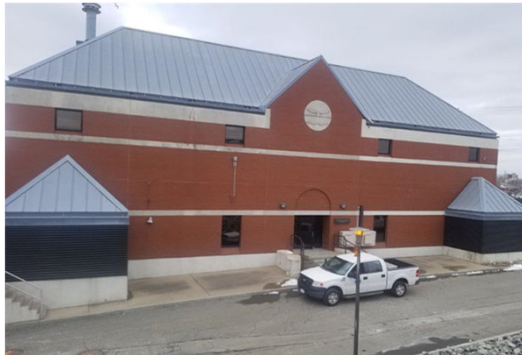
Photo: Ernest Street Pump Station
