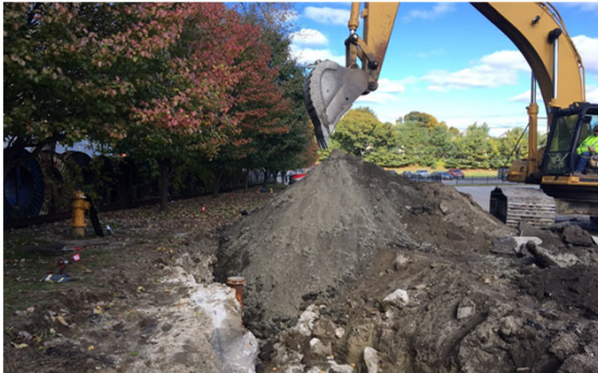
Photo: Construction on the Moshassuck Valley Interceptor
