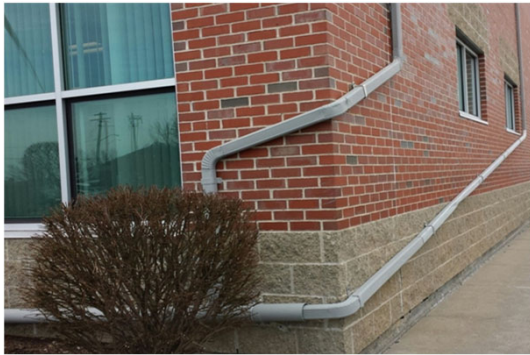
Photo: Downspouts at NBC's Corporate Office Building
