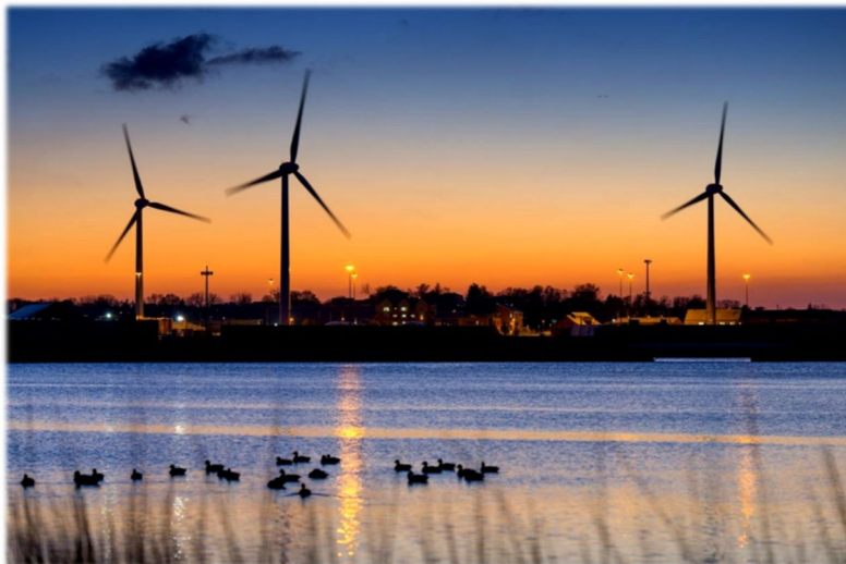
Photo: Sunset over Field’s Point Wastewater Treatment Facility Wind Turbines Providence River, Rhode Island
