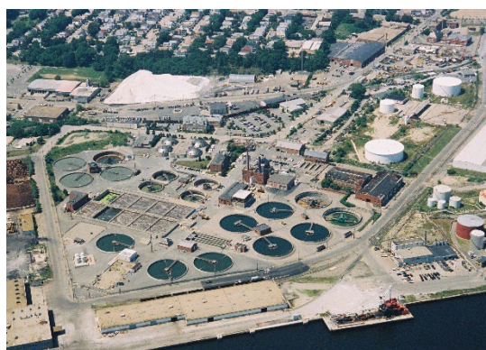
Field's Point Wastewater Treatment Facility
