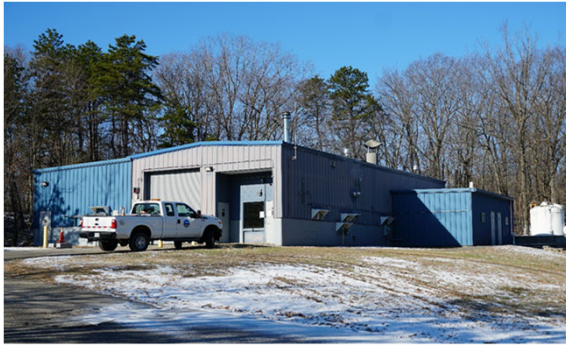
Photo: Lincoln Septage Receiving Station
