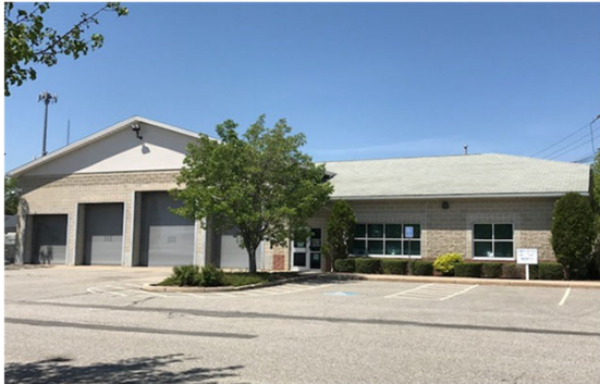
Photo: Interceptor Maintenance Building
