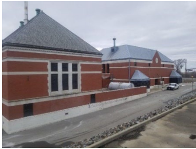
FPWWTF Ernest Street Pump Station
