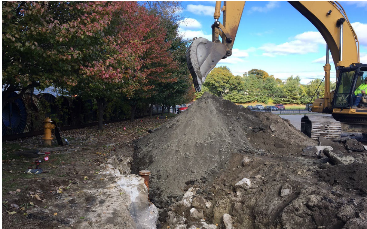
Photo: Construction on the Moshassuck Valley Interceptor
