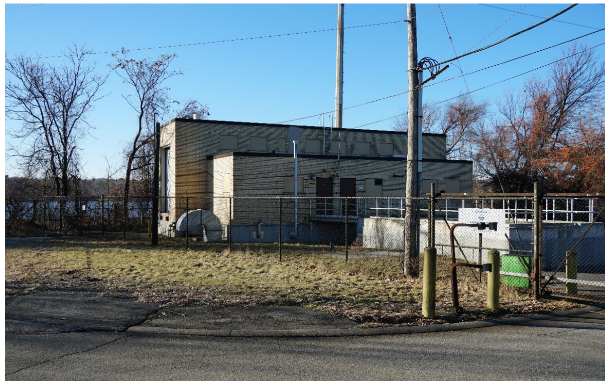
Photo: Omega Pump Station
