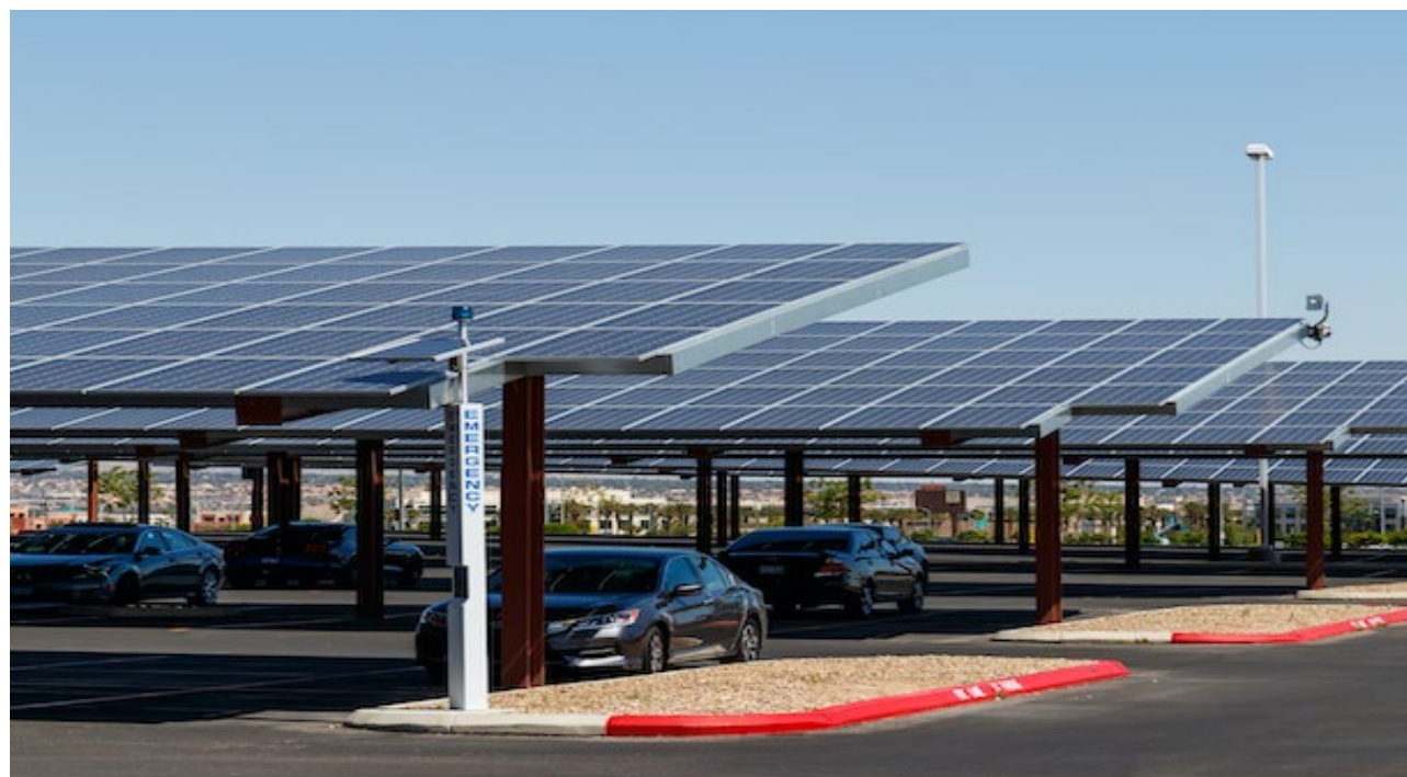
Photo: Solar Carport
