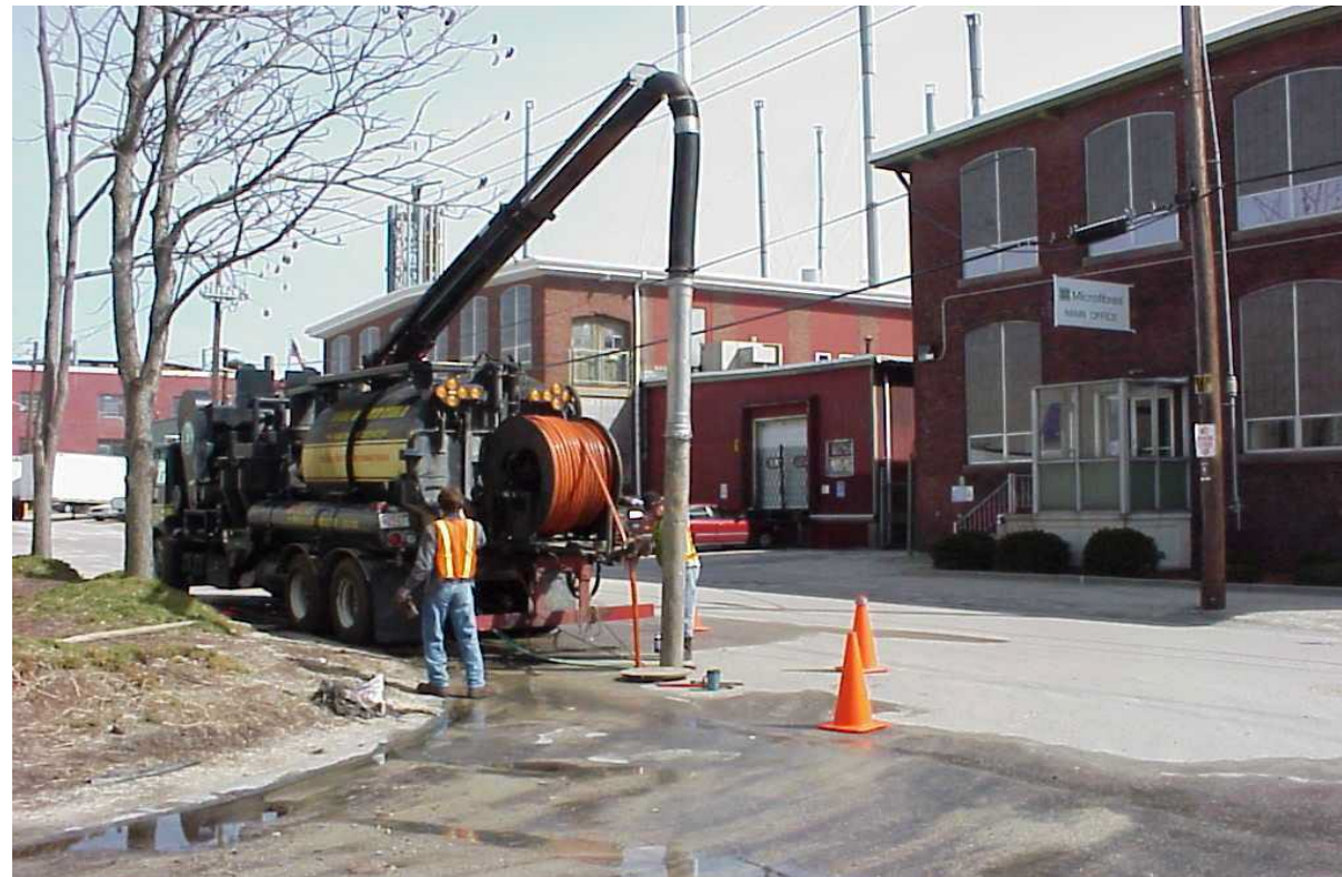
Photo: Interceptor Grit Removal
