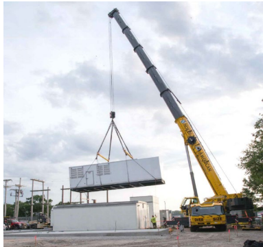
Photo: 2,000 kWh Generator Installation
