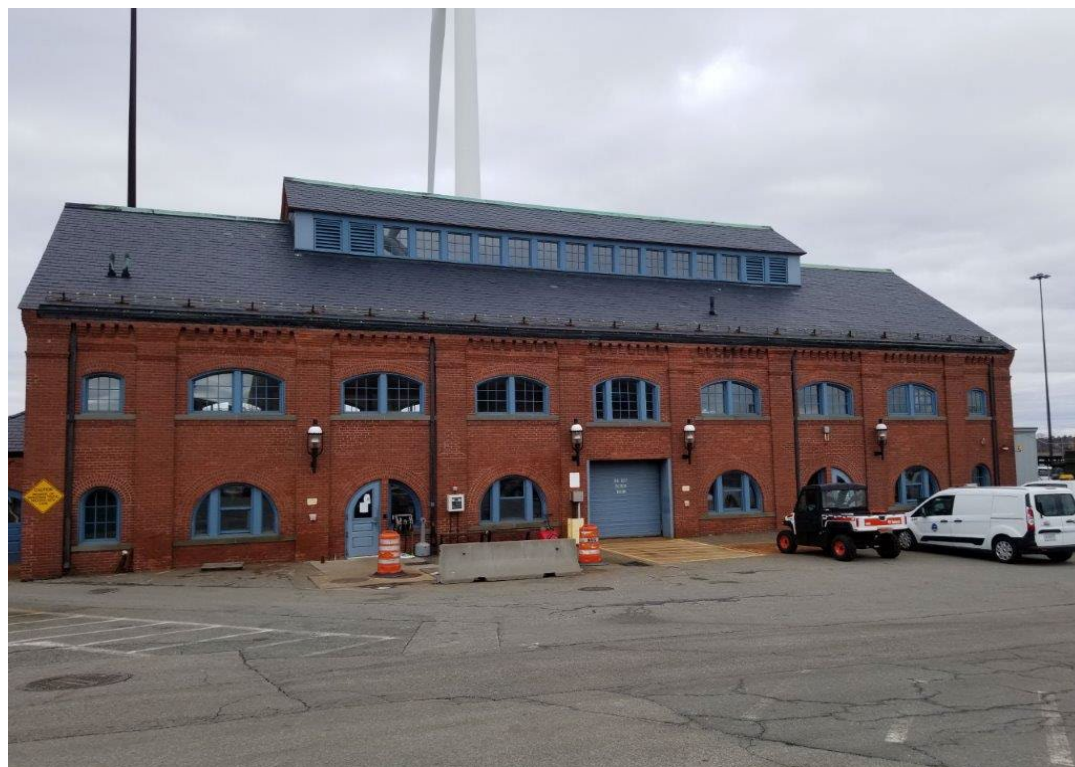
Photo: Existing FPWWTF Maintenance Building
