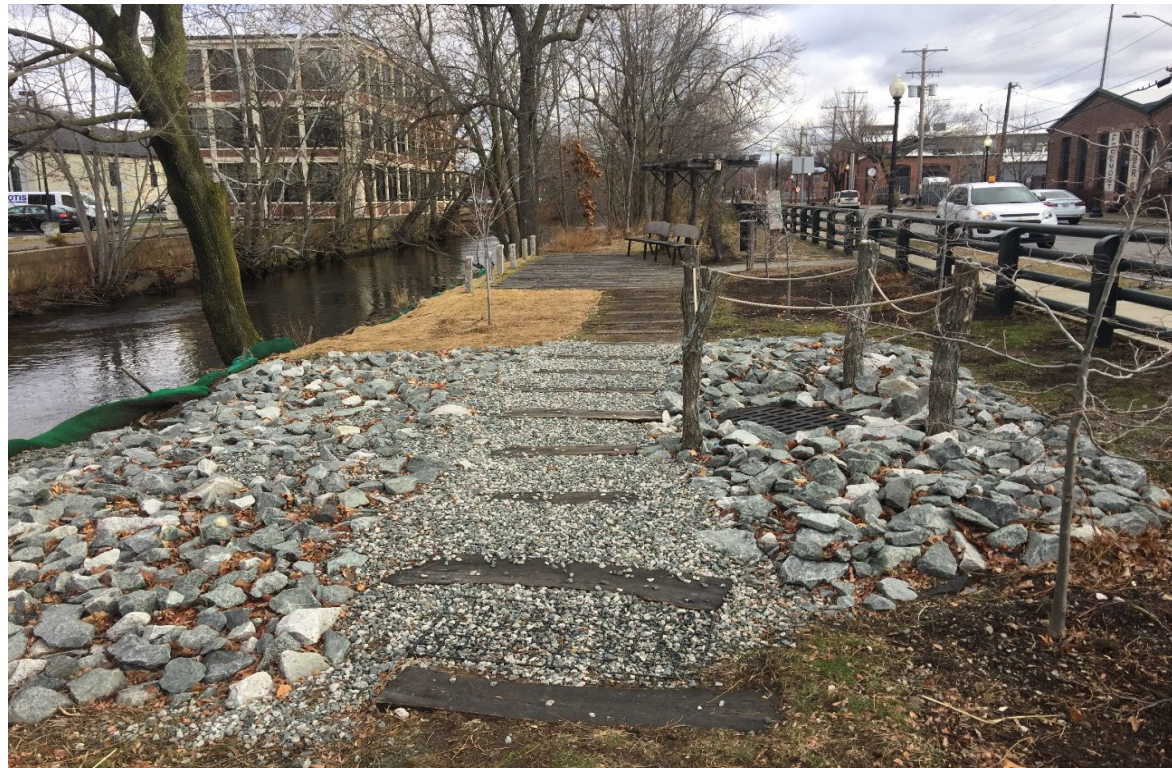
Photo: Proposed portion of Lincoln Interceptor Replacement
