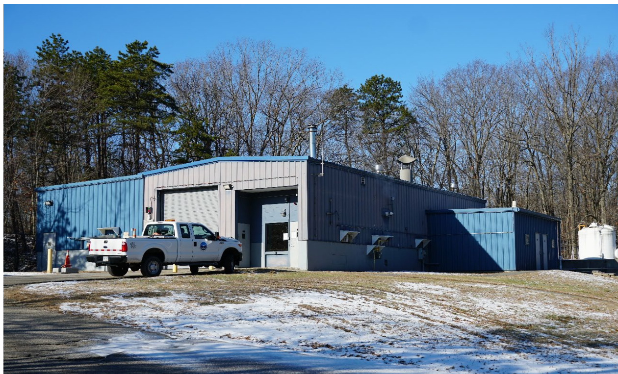
Photo: Lincoln Septage Receiving Station
