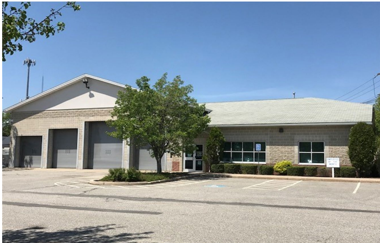
Photo: Interceptor Maintenance Building
