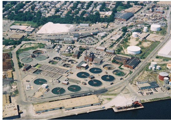
Field's Point Wastewater Treatment Facility
