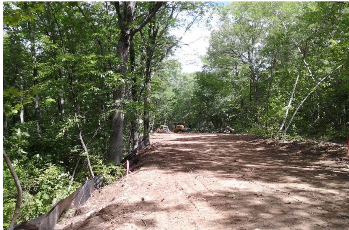
Photo: Easement Clearing
