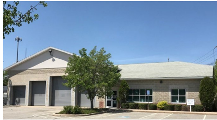
Interceptor Maintenance Building
