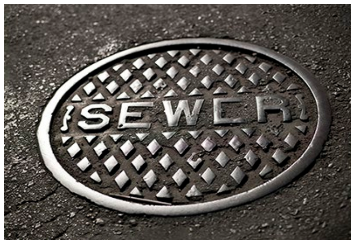
Photo: Municipal Sewer Manhole Cover
