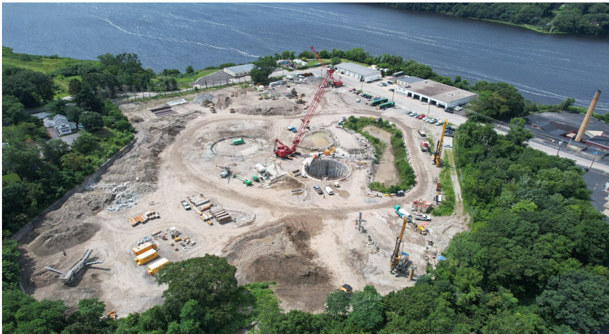
Photo: Pawtucket Tunnel Site
