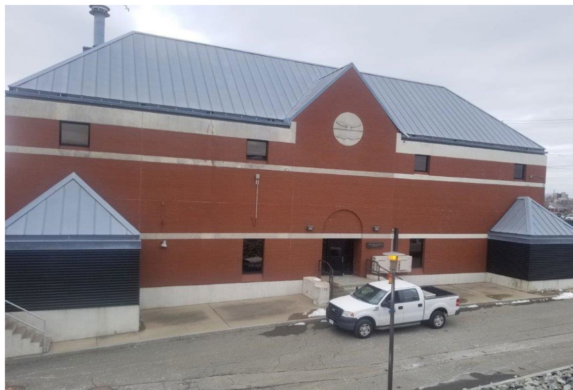
Photo: Ernest Street Pump Station
