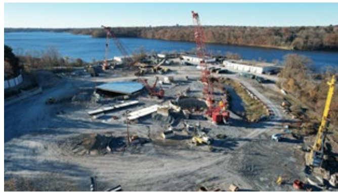
Pawtucket Tunnel Pump Station Site
