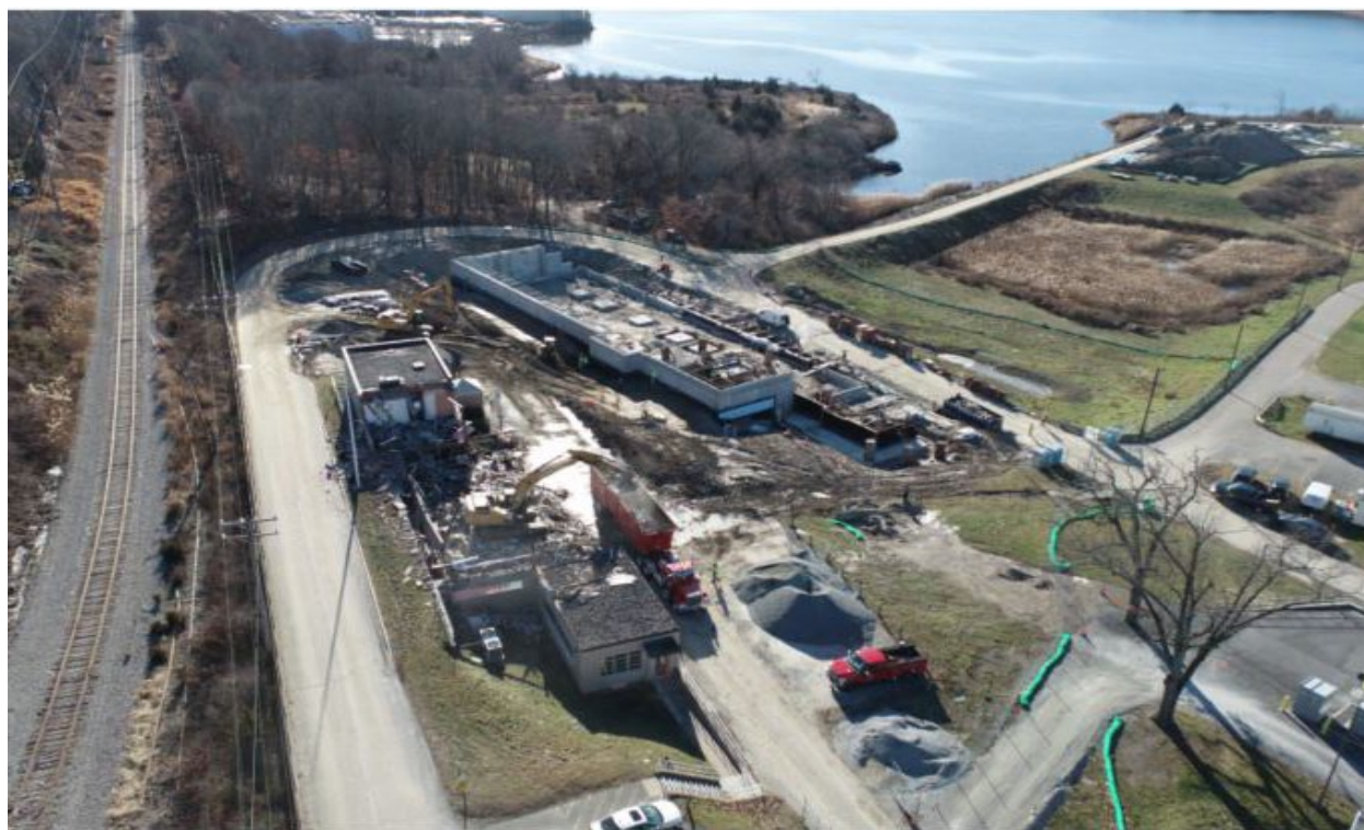
Photo: Operations & Maintenance Building
