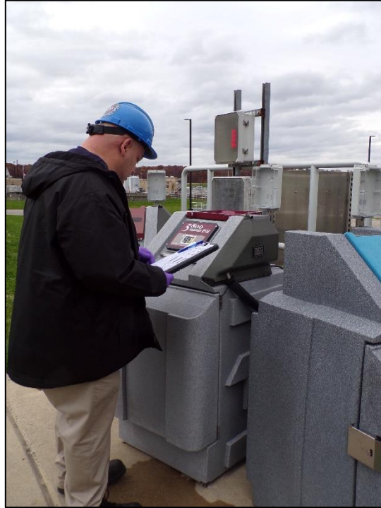
Environmental monitor records data at the Bucklin Point WWTF.
