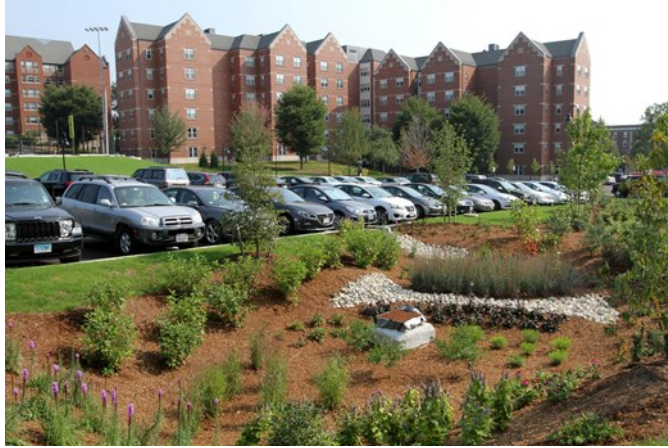
These areas are graded to divert excess runoff away from the building.
