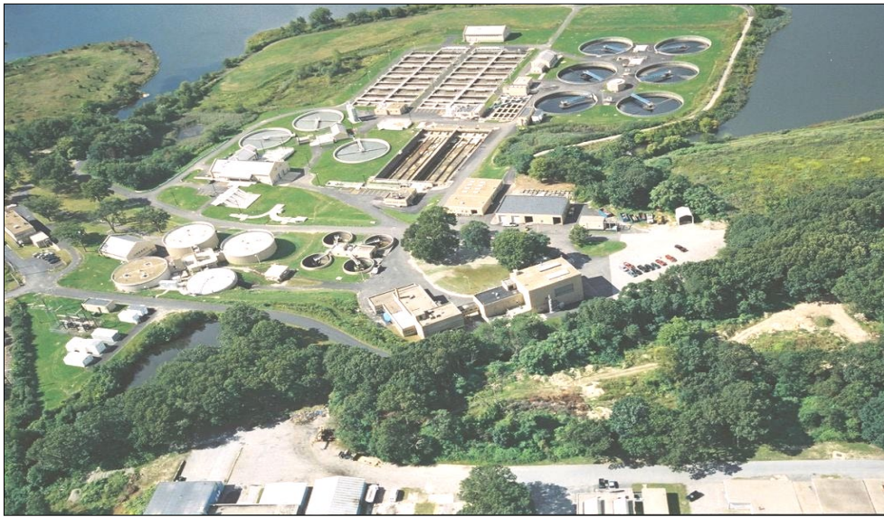
Bucklin Point Wastewater Treatment
