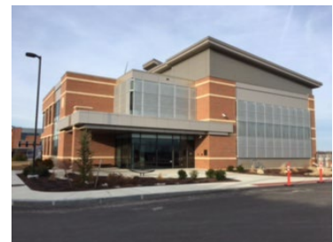
Water Quality Science Building
