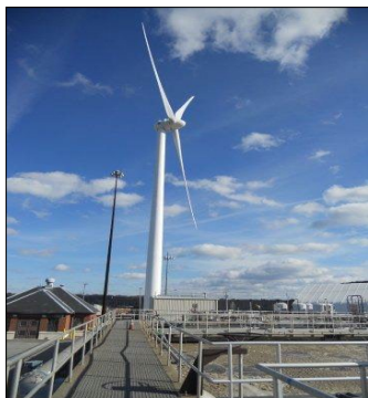
Field's Point Wind Turbine and IFAS Tank
