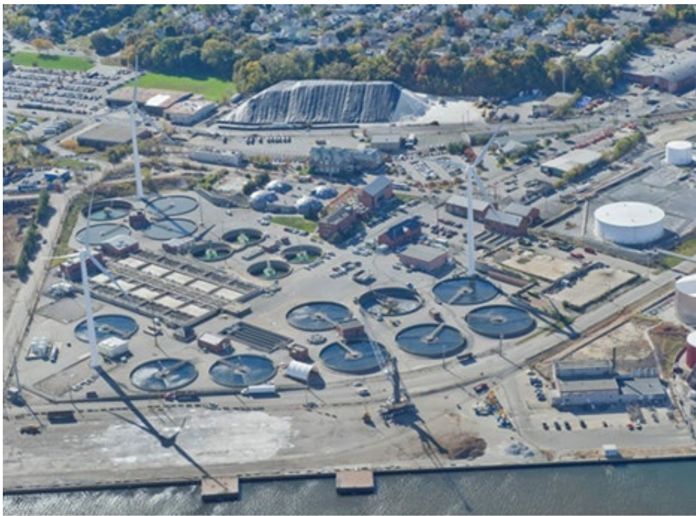
Field's Point Wastewater Treatment Facility
