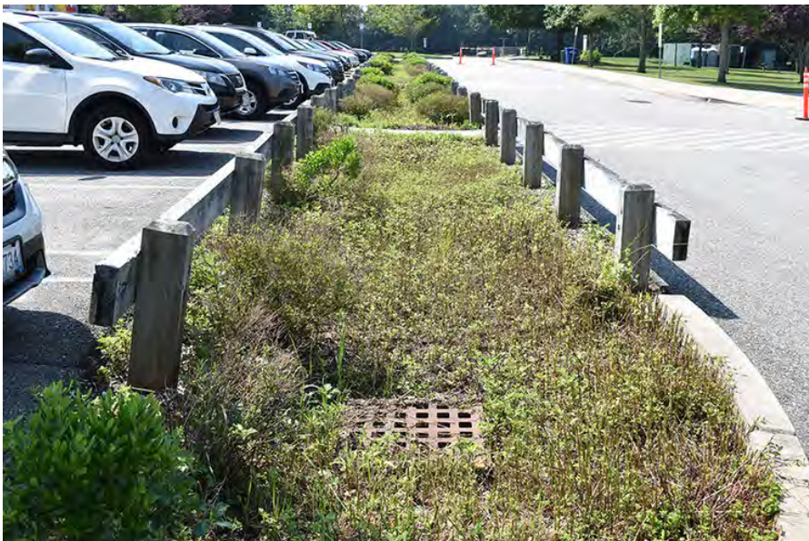
Bioretention rain gardens in the parking lot of Bristol Town Beach have helped reduce the amount of stormwater that reaches the beach unfiltered. (Frank Carini/ecoRI News)
