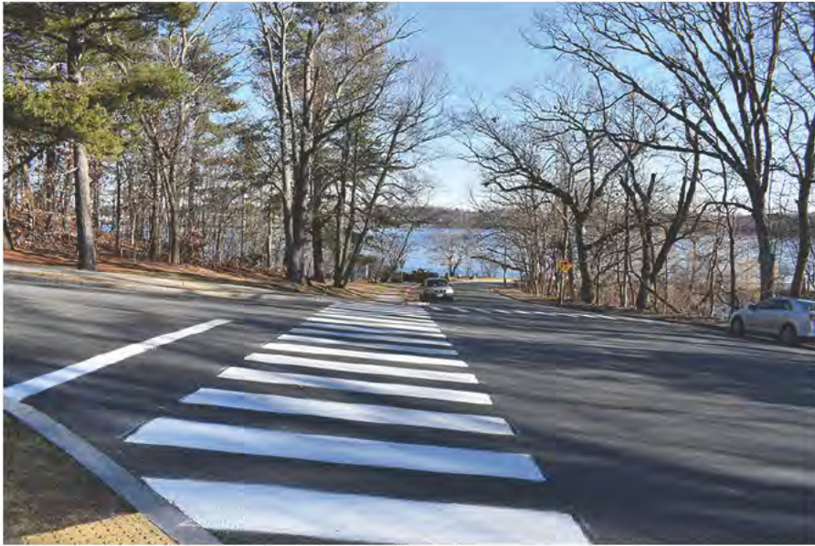
This expanse of asphalt at the intersection of Irving Avenue and Loring Avenue on Providence's East Side drives stormwater runoff to the banks of the Seekonk River.
