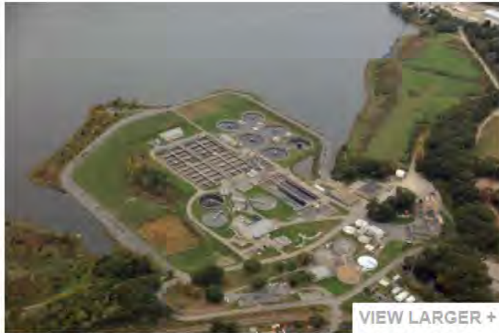
Bucklin Point Wastewater Treatment Facility, PHOTO: NBC
