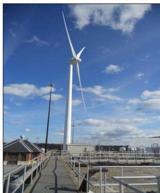
Field's Point Wind Turbine
