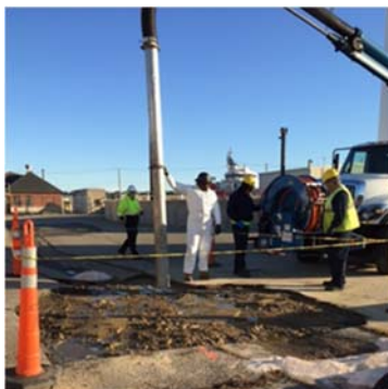
Sodium Hypochlorite Spill & Repair
