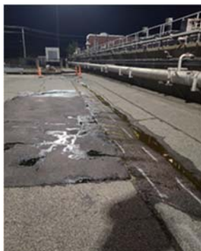
Sodium Hypochlorite Spill & Repair
