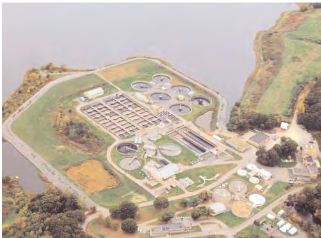
Bucklin Point Aerial Shot.
