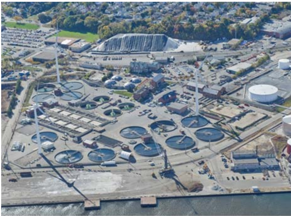
Field's Point Wastewater Treatment Facility
