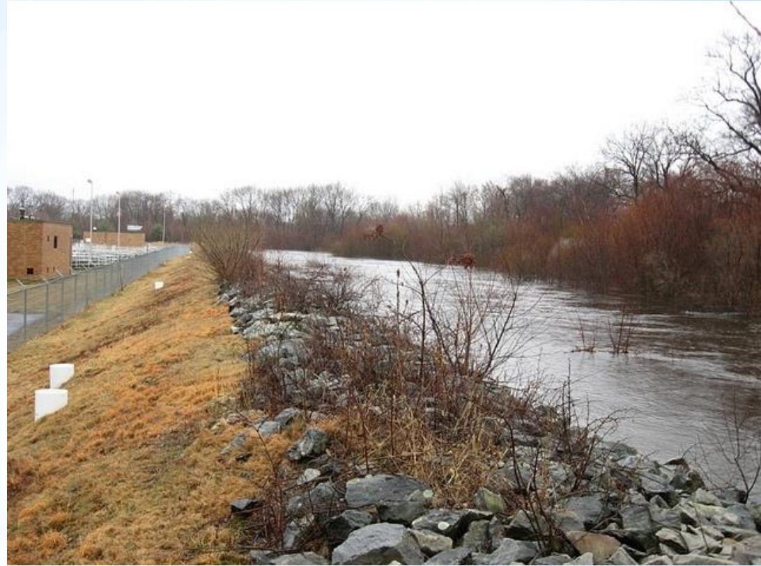
Warwick WWTF Berm Designed for 100 Year Storm
