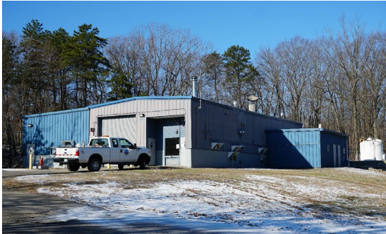
Photo: Lincoln Septage Receiving Station
