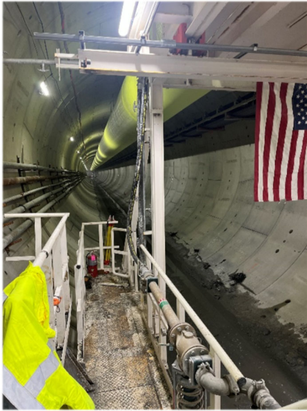
Inside the Pawtucket deep rock tunnel - Project 30801
