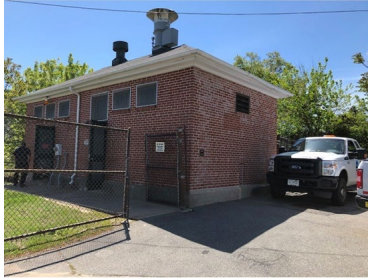
Reservoir Avenue Pump Station
