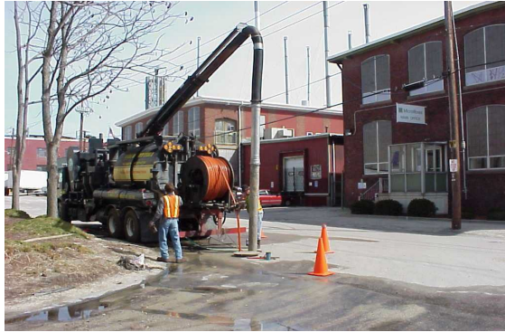
Photo: Interceptor Grit Removal
