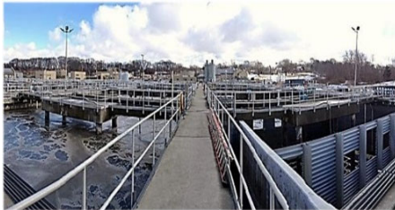
Aeration Tanks at the Field's Point Wastewater Treatment Facility
