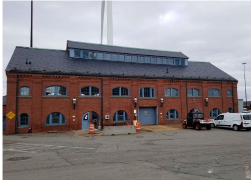
Photo: Existing FPWWTF Maintenance Building
