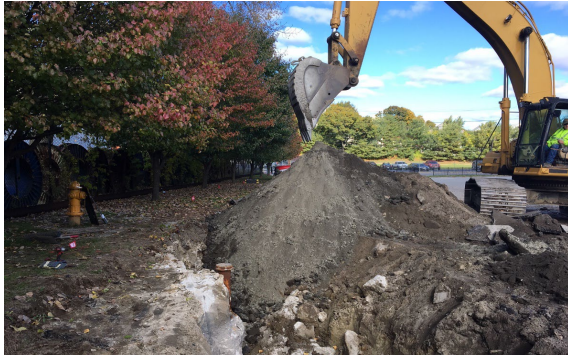
Photo: Construction on the Moshassuck Valley Interceptor
