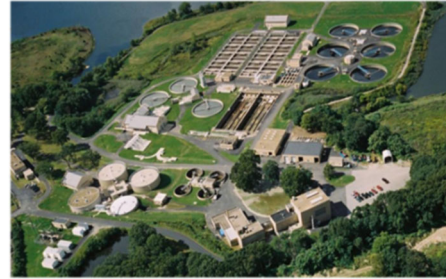
Bucklin Point Wastewater Treatment Facility
