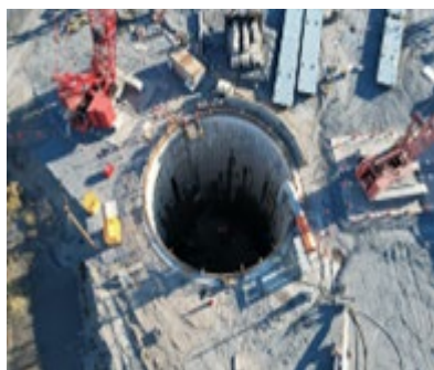
Photo: CSO Phase III A Facilities Pawtucket Tunnel
