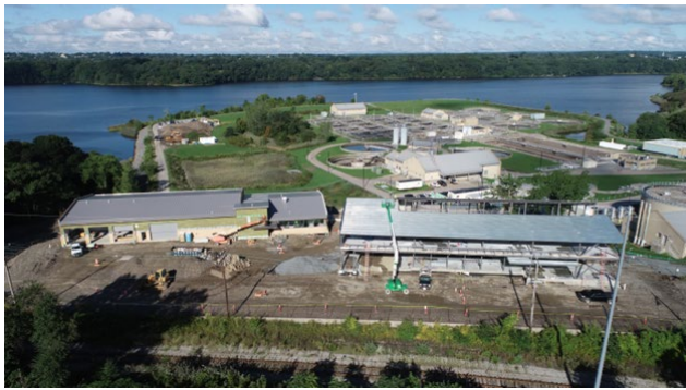
New BPWWTF Operations and Maintenance Buildings
