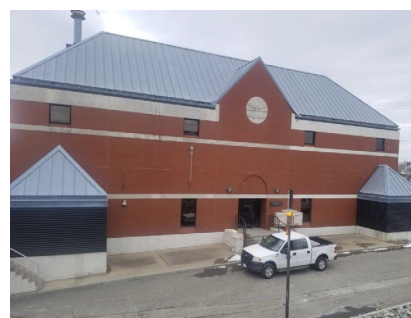
FPWWTF Ernest Street Pump Station
