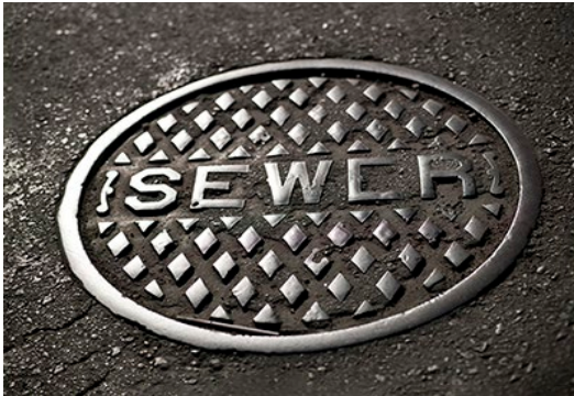
Photo: Municipal Sewer Manhole Cover
