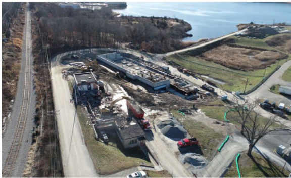
Photo: Operations and Maintenance Building
