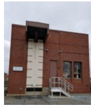
Field’s Point Primary Sludge Pump Station
