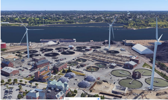
Photo: Aerial of the FPWWTF and the Providence River
