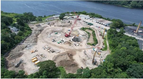
Photo: Pawtucket Tunnel Site
