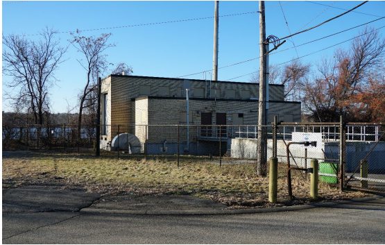
Photo: Omega Pump Station
