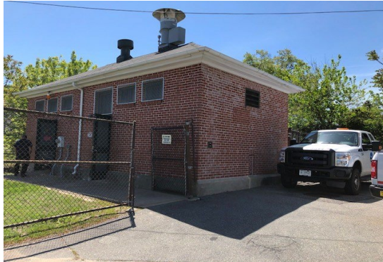
Photo: Reservoir Avenue Pump Station
