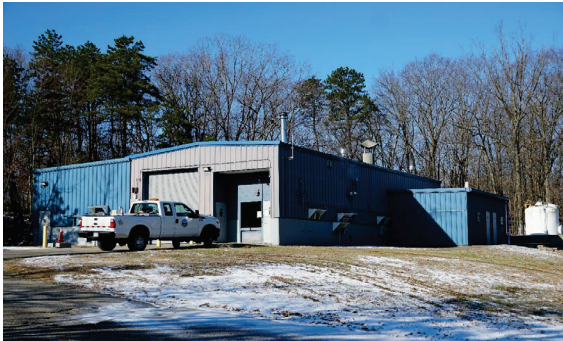
Photo: Lincoln Septage Receiving Station
