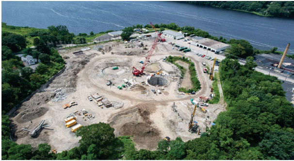
Photo: Pawtucket Tunnel Site
