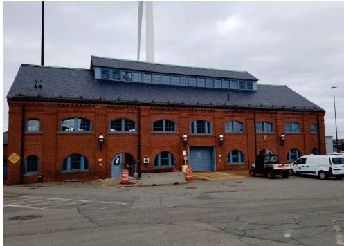
Photo: Existing FPWWTF Maintenance Building
