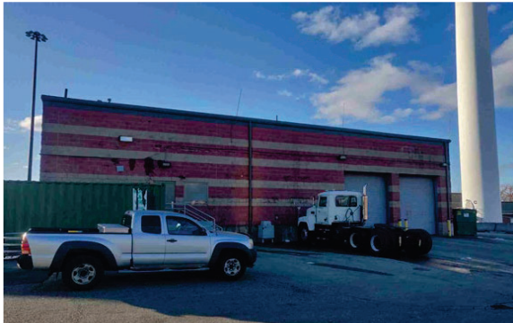
Photo: Sludge Dewatering and Handling Facility
