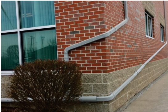
Photo: Downspouts at NBC's Corporate Office Building
