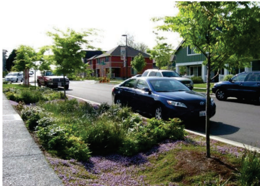
Photo: Example of Green Stormwater Infrastructure
