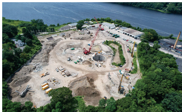
CSO Phase III A Pawtucket Tunnel Pump Station Site
