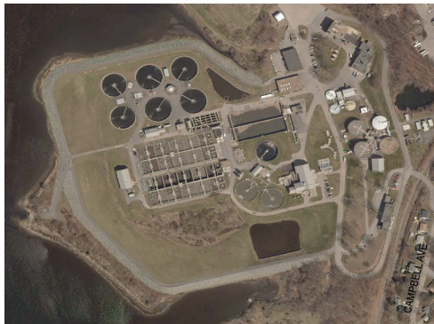
Photo: Existing Clarifiers at Bucklin Point
