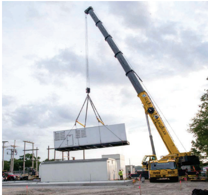
Photo: 2,000 kWh Generator Installation
