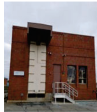
Field's Point Primary Sludge Pump Station
