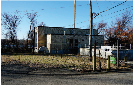
Photo: Omega Pump Station
