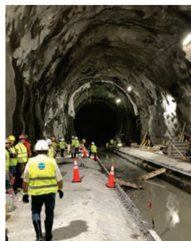
CSO Tunnel Construction
