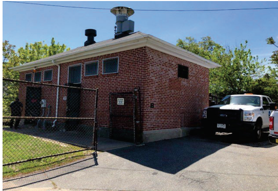
Photo: Reservoir Avenue Pump Station
