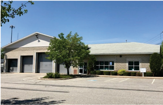
Photo: Interceptor Maintenance Building
