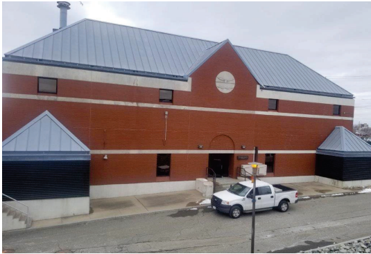
Photo: Ernest Street Pump Station
