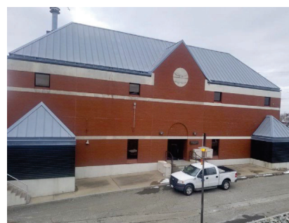
FPWWTF Ernest Street Pump Station
