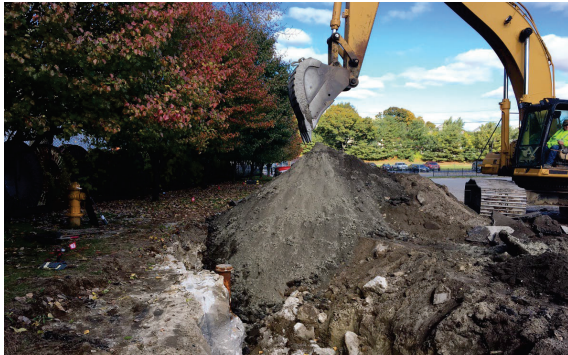
Photo: Construction on the Moshassuck Valley Interceptor
