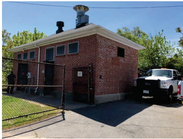
Reservoir Avenue Pump Station
