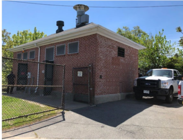
Reservoir Avenue Pump Station
