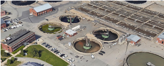
Photo: Wet Weather Clarifiers
