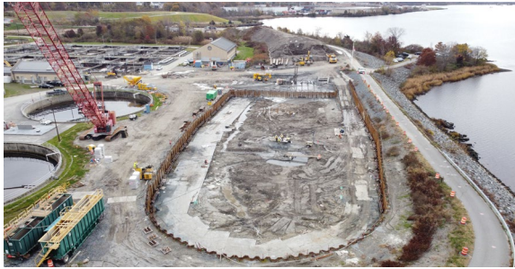
Photo: Construction Underway - Clarifiers at Bucklin Point
