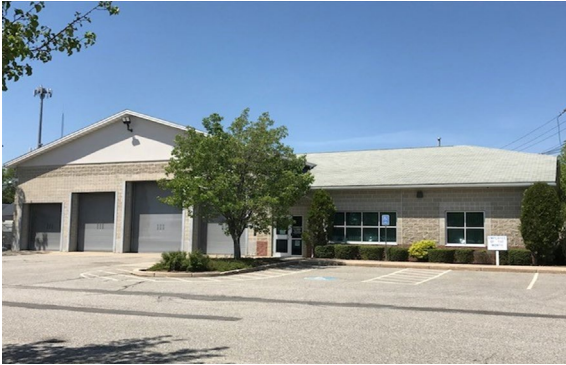
Photo: Interceptor Maintenance Building
