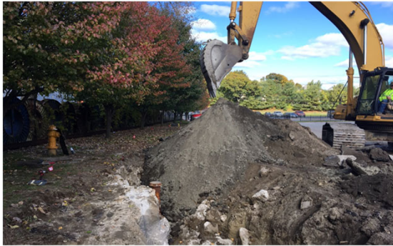
Photo: Construction on the Moshassuck Valley Interceptor
