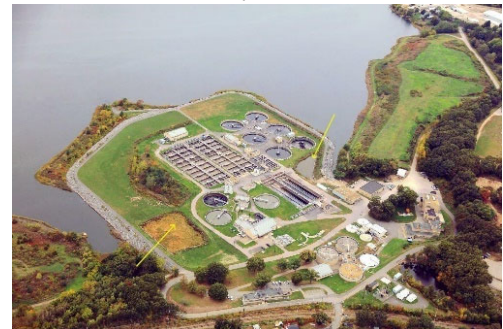
Bucklin Point Wastewater Treatment Facility
