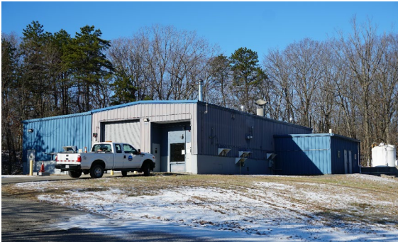
Photo: Lincoln Septage Receiving Station
