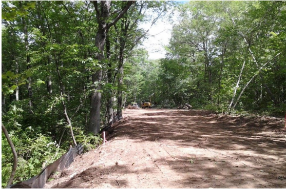
Photo: Easement Clearing
