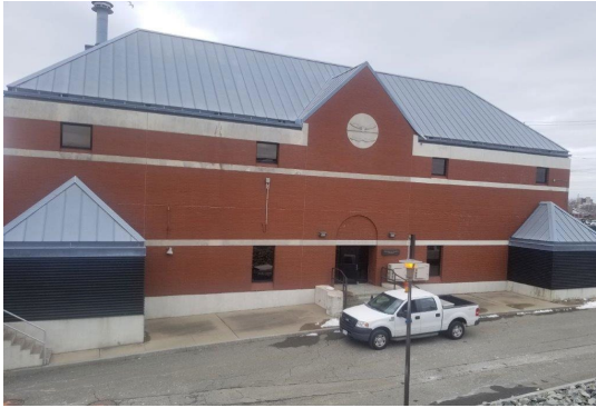
Photo: Ernest Street Pump Station
