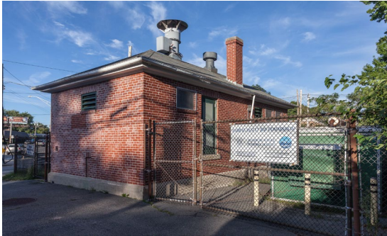
Photo: Reservoir Avenue Pump Station
