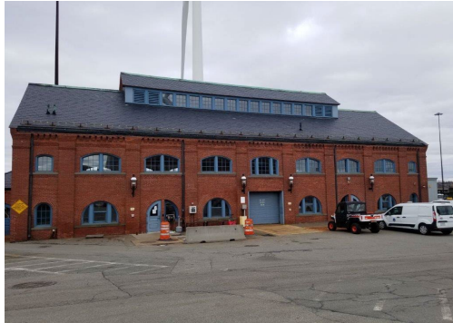
Photo: Existing FPWWTF Maintenance Building
