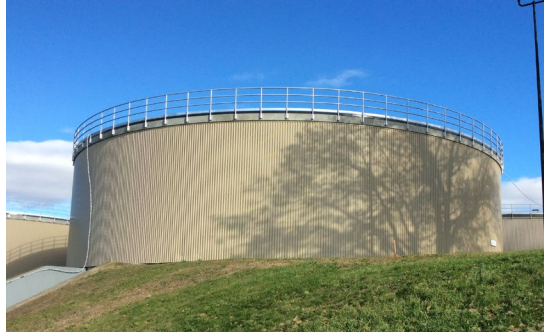
Photo: Bucklin Point Digester
