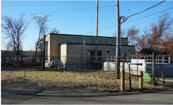
Photo: Omega Pump Station
