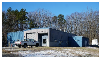
Lincoln Septage Receiving Station
