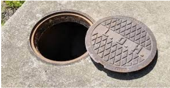
Photo: Municipal Sewer Manhole Cover
