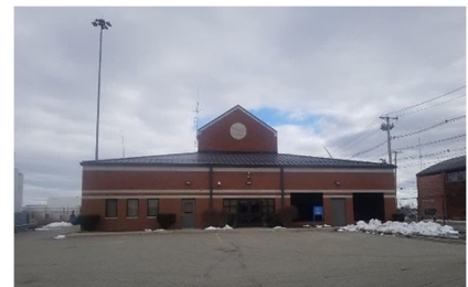
FPWWTF Ernest Street Pump Station
