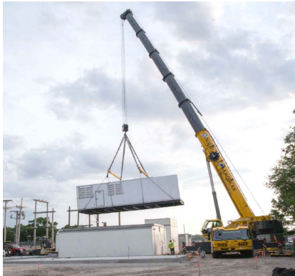
Photo: 2,000 kWh Generator Installation
