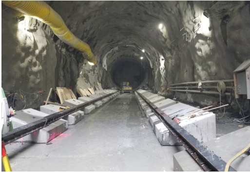
Photo: Pawtucket Tunnel Site
