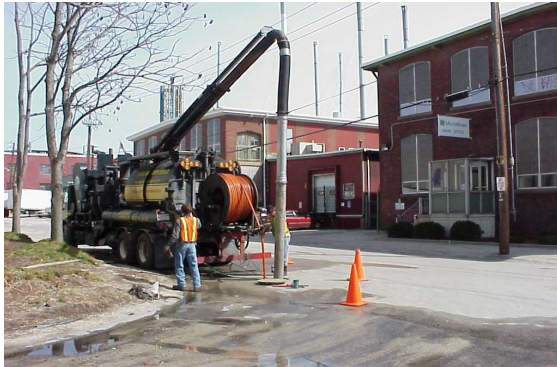
Photo: Interceptor Grit Removal
