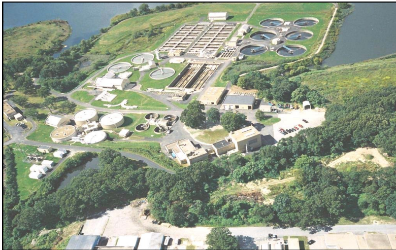
Aerial view of the Bucklin Point WWTF
