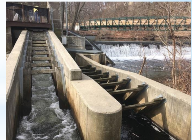
Fish ladder, Manton Dam, Woonasquatucket River.
