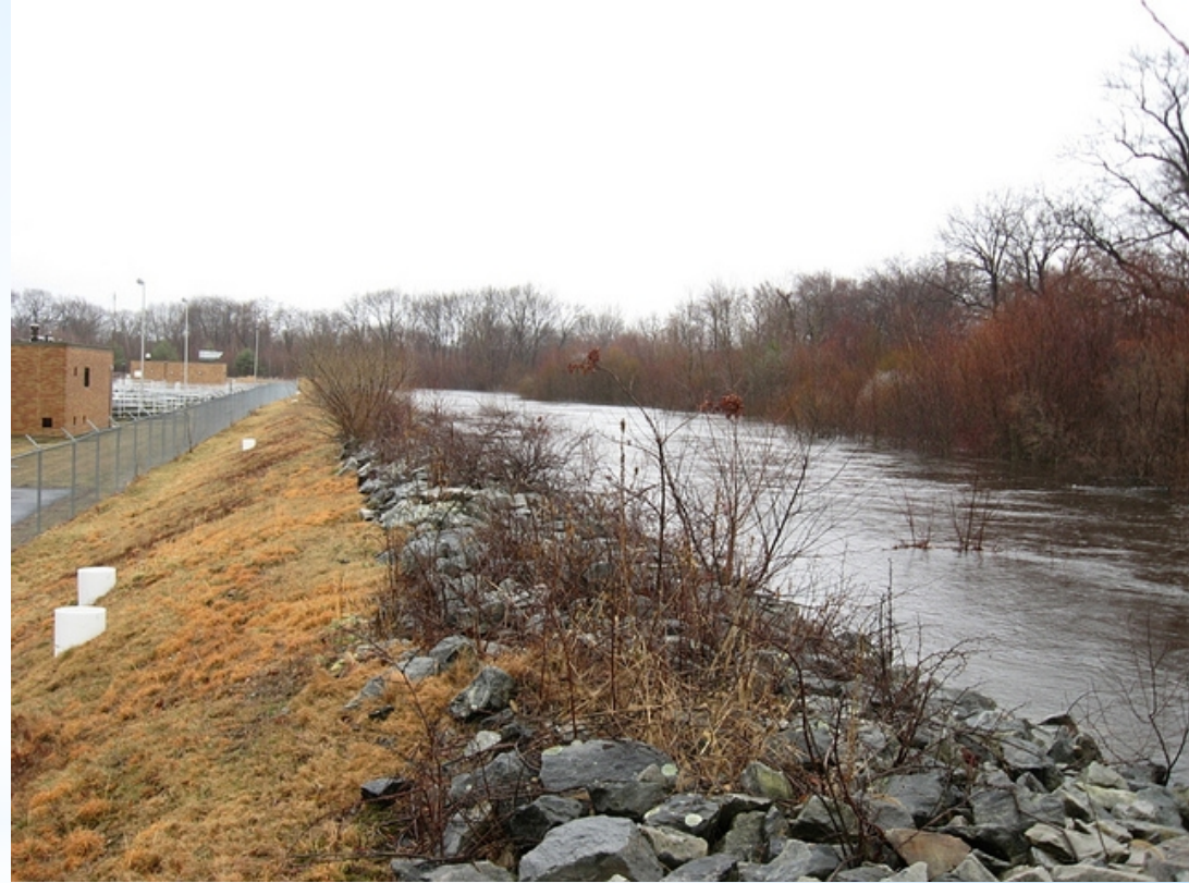
Warwick WWTF Berm Designed for 100 Year Storm
