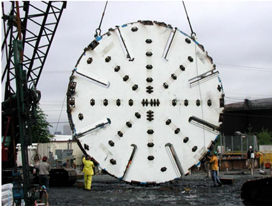
Figure 1. Cutter head of the 30 ft. diameter Tunnel Boring Machine (TBM)
