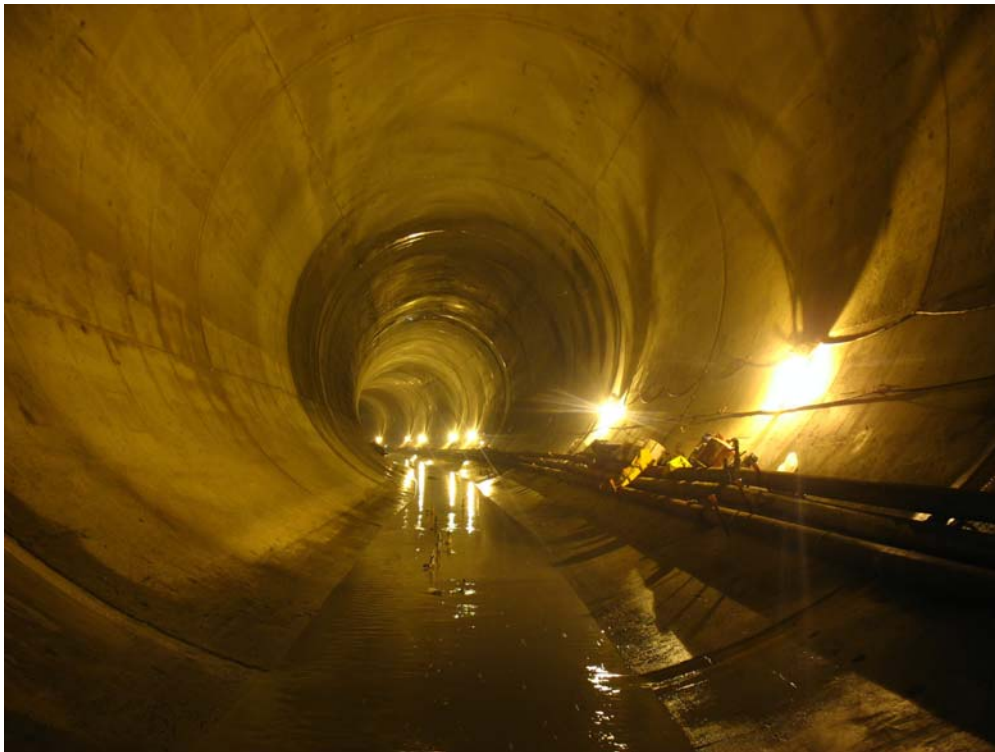
Figure 5. Completed 26 foot diameter tunnel
