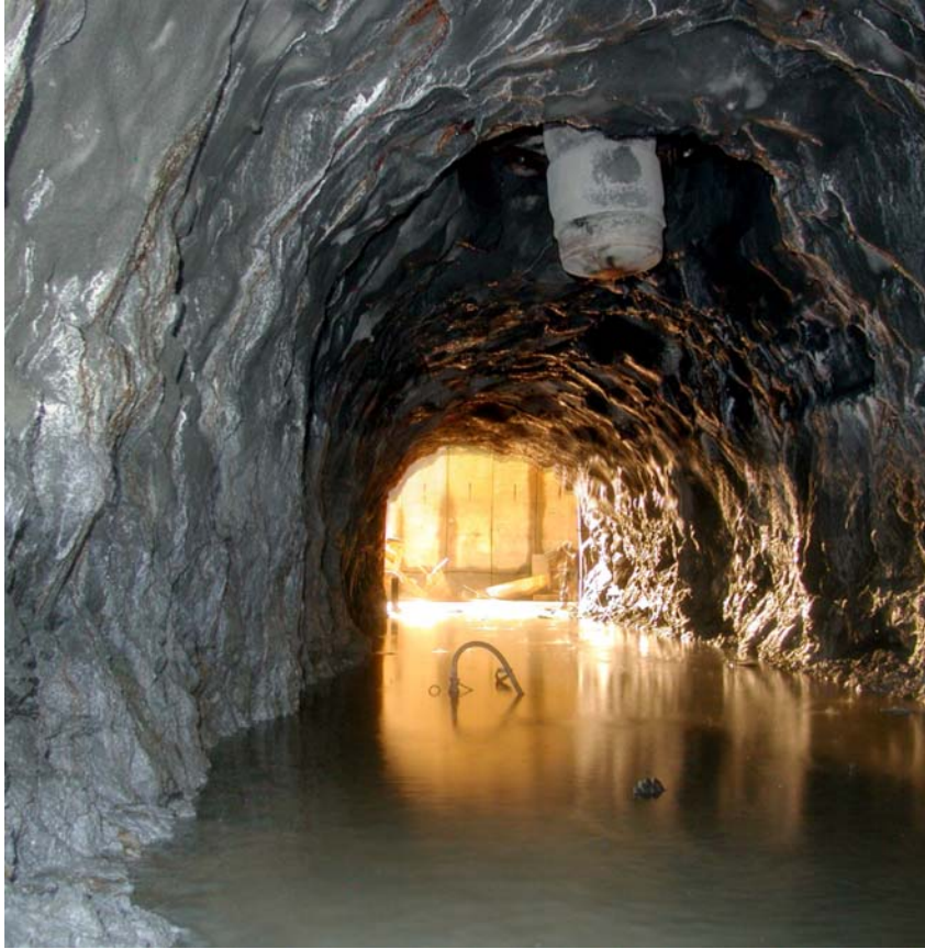
Figure 2. Mined drop shaft adit looking towards entrance into tunnel
