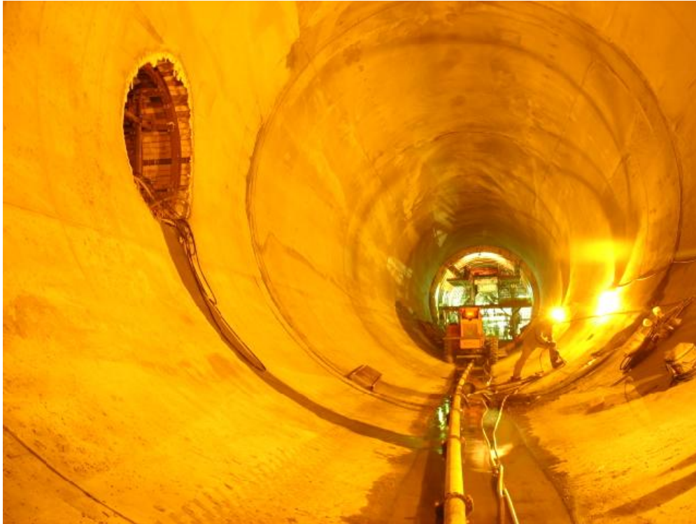
Figure 3. Nearly completed adit (on left) into tunnel
