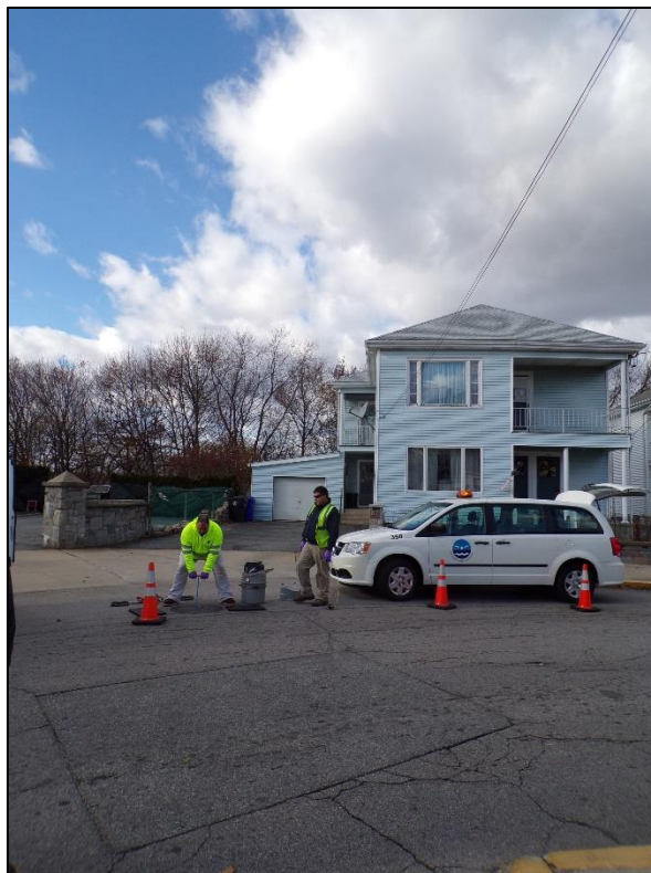
Environmental monitors conduct sanitary manhole sampling.
