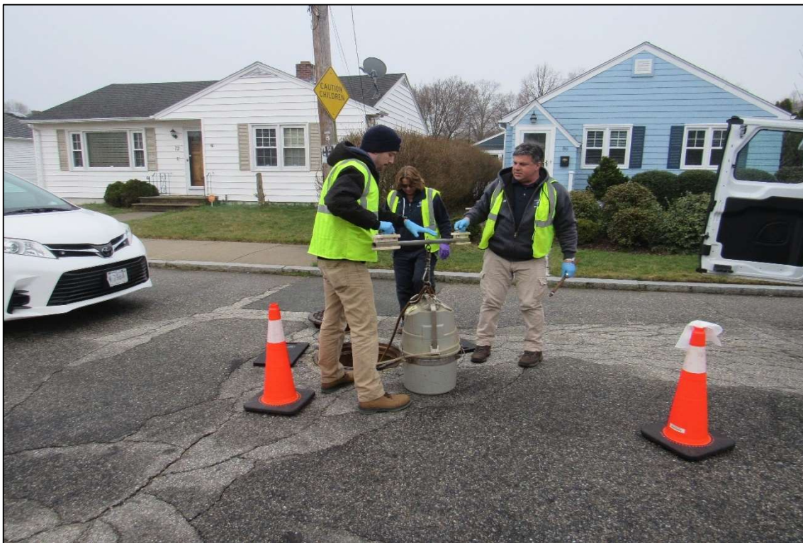
Environmental monitors conduct sanitary manhole sampling.
