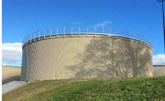
Photo: Bucklin Point Digester
