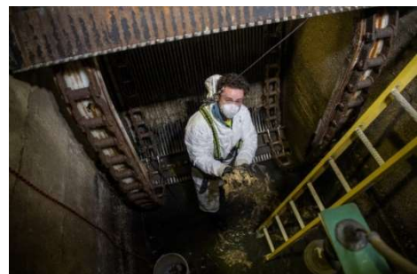
Debris removal in Screening & Grit Photo by Peter Goldberg
