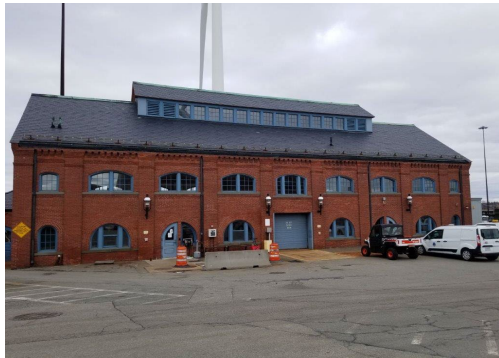
Photo: Existing FPWWTF Maintenance Building
