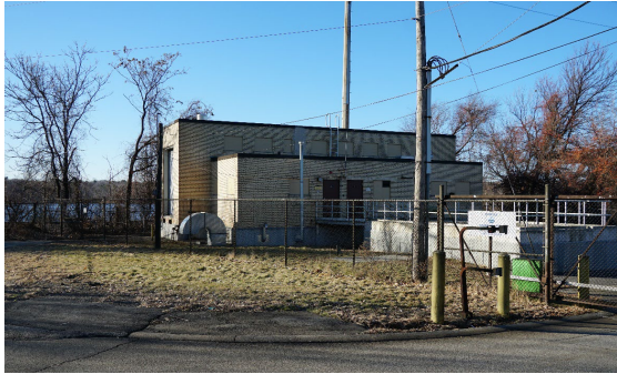
Photo: Omega Pump Station
