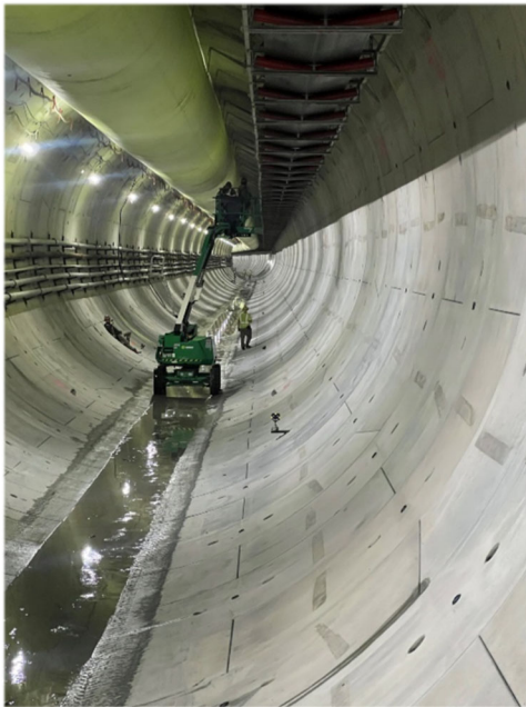
Inside the Pawtucket deep rock tunnel - Project 30801
