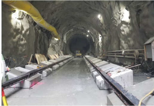
Photo: Pawtucket Tunnel Site
