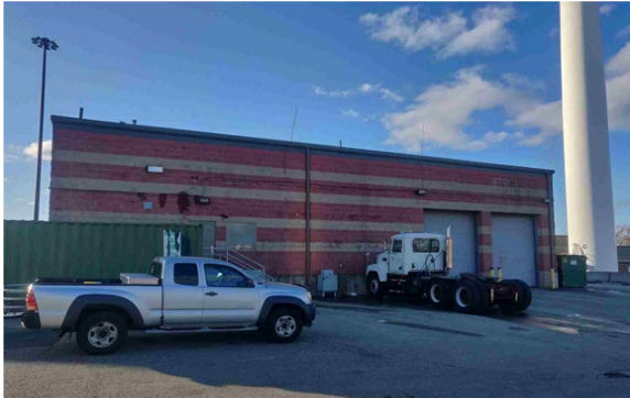
Photo: Sludge Dewatering and Handling Facility
