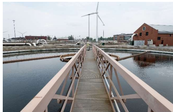
Catwalk over Secondary Treatment Final Clarifier Tank Photo by Peter Goldberg
