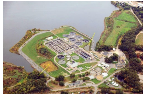
Bucklin Point Wastewater Treatment Facility
