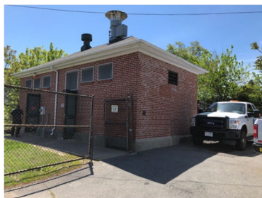
Reservoir Avenue Pump Station
