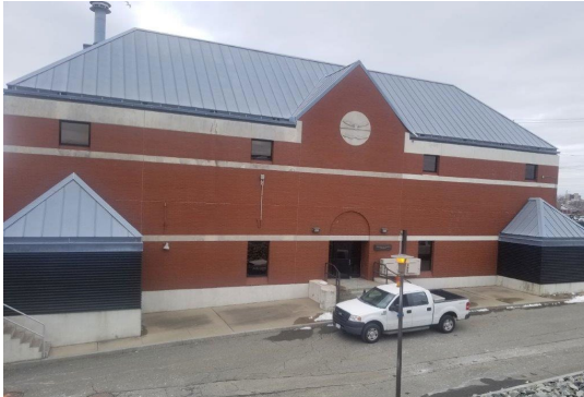
Photo: Ernest Street Pump Station
