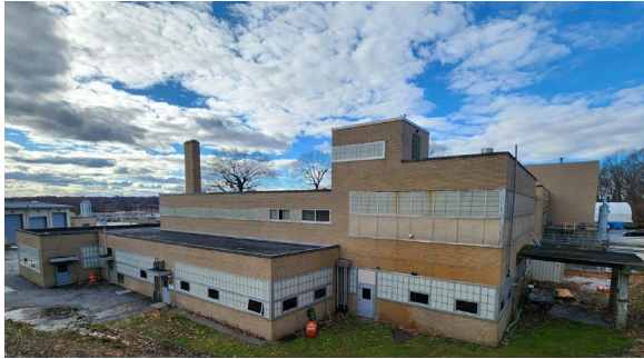
Photo: Bucklin Point Operations Building
