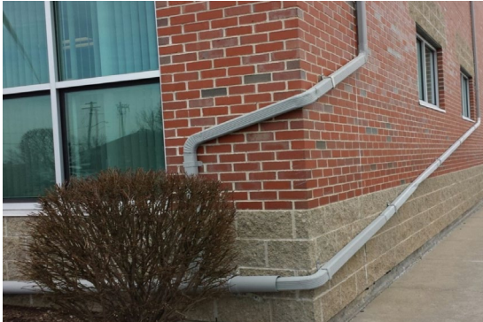
Photo: Downspouts at NBC's Corporate Office Building
