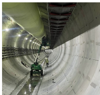
Photo: CSO Phase III A Facilities Pawtucket Tunnel
