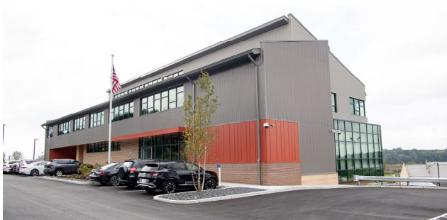
New Bucklin Point Wastewater Treatment Facility Operations Building – Photo by Peter Goldberg
