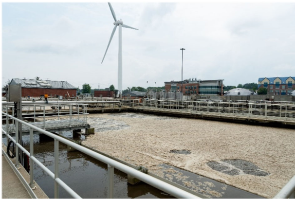
Aeration Tanks at Field's Point WWTF Photo by Peter Goldberg
