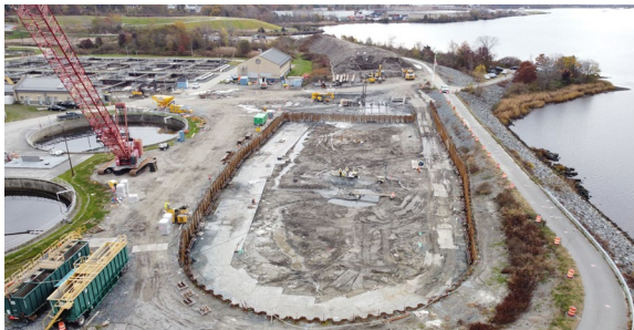
Photo: Construction Underway - Clarifiers at Bucklin Point
