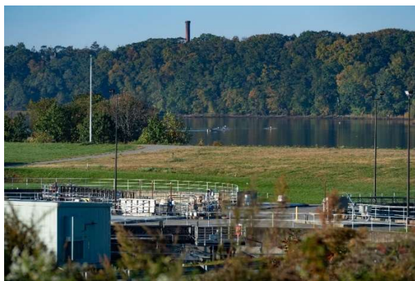
Seekonk River from Bucklin Point WWTF Photo by Peter Goldberg
