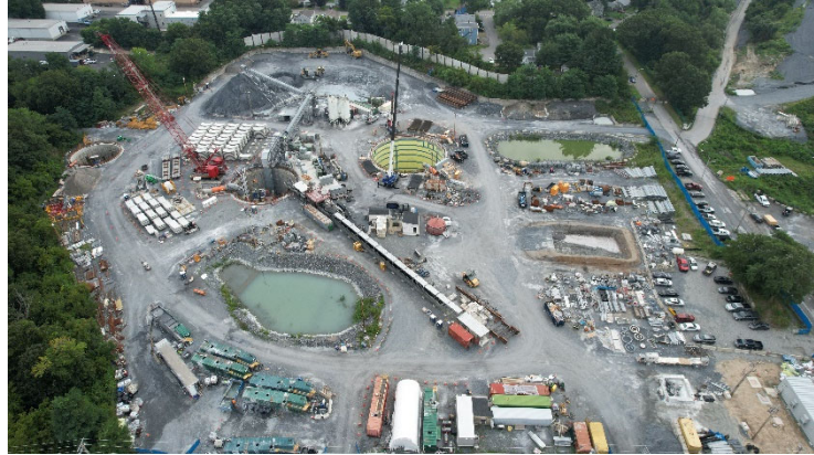
CSO Phase III A Pawtucket Tunnel and Pump Station Shaft Construction Site
