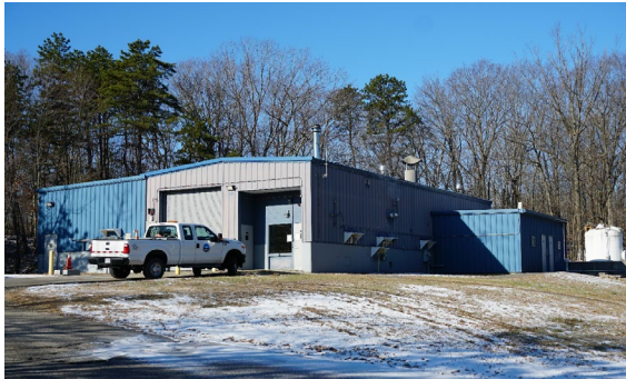
Photo: Lincoln Septage Receiving Station
