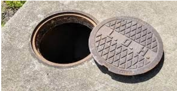
Photo: Municipal Sewer Manhole Cover
