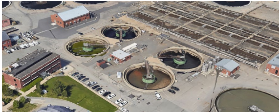
Photo: Wet Weather Clarifiers
