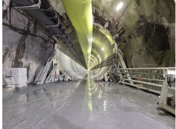
CSO Phase III A Tunnel Construction
