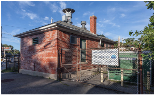
Photo: Reservoir Avenue Pump Station
