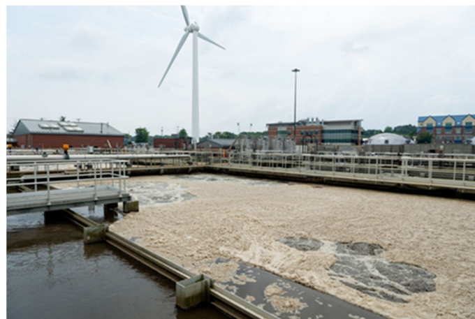
Integrated Fixed Film Activated Sludge (IFAS) Tank Photo by Peter Goldberg
