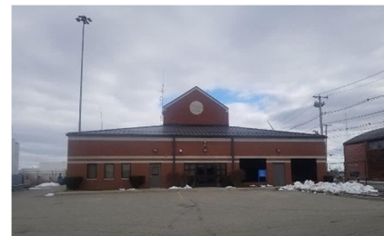
FPWWTF Ernest Street Pump Station
