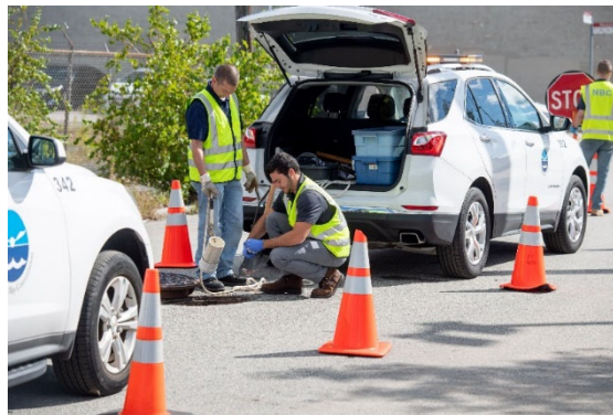
Investigation of Influent in Manhole Photo by Peter Goldberg
