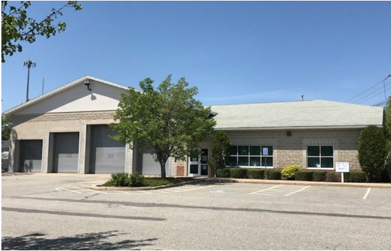
Photo: Interceptor Maintenance Building
