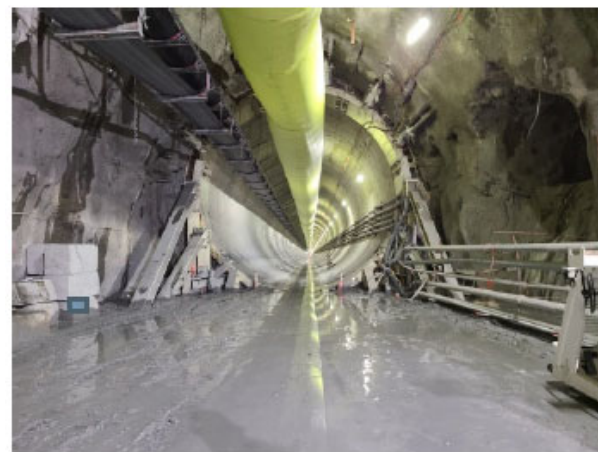
CSO Phase III A Tunnel Construction
