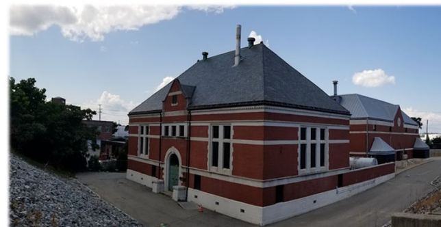
Ernest Street Pumping Station
