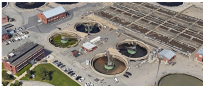
Field's Point Wet Weather Clarifiers
