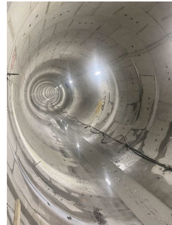
CSO Phase III A Tunnel Construction
