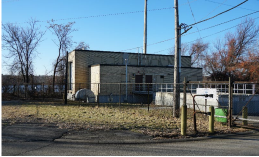
Photo: Omega Pump Station
