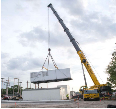
Photo: 2,000 kWh Generator Installation
