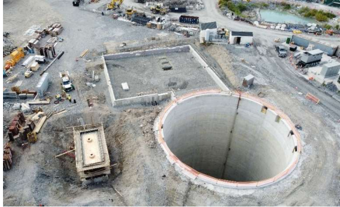
CSO Phase III A Pawtucket Tunnel Pump Station Fit-Out Construction Site
