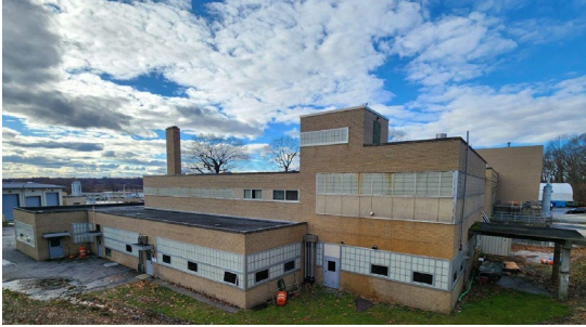
Photo: Bucklin Point Operations Building
