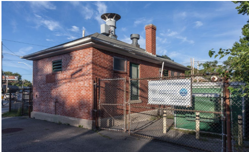
Photo: Reservoir Avenue Pump Station
