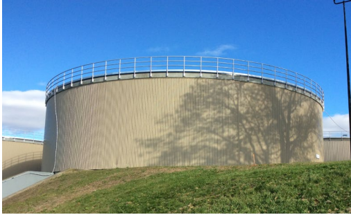
Photo: Bucklin Point Digester
