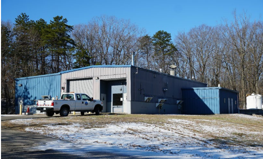
Photo: Lincoln Septage Receiving Station
