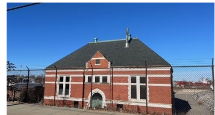
FPWWTF Ernest Street Pump
