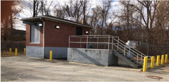
Photo: Saylesville Pump Station
