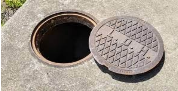
Photo: Municipal Sewer Manhole Cover
