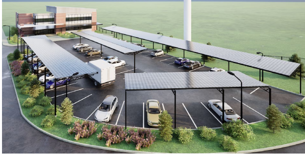
Photo: Solar Carport
