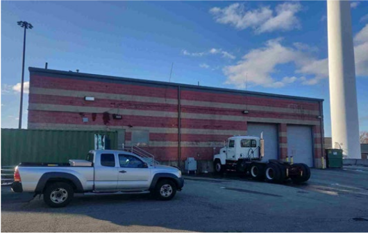
Photo: Sludge Dewatering and Handling Facility
