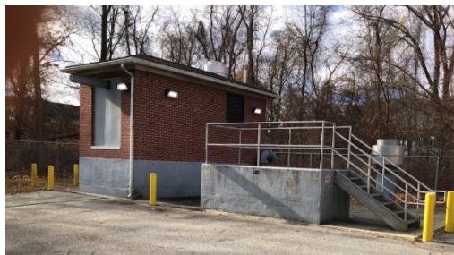
Saylesville Pump Station
