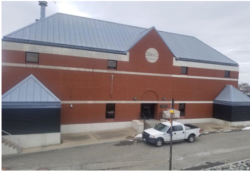
Photo: Ernest Street Pump Station
