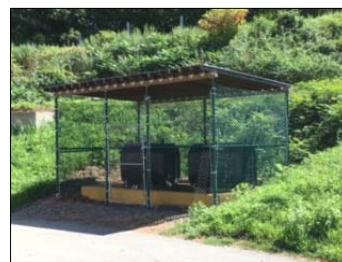
Used Oil Storage Containment Area
