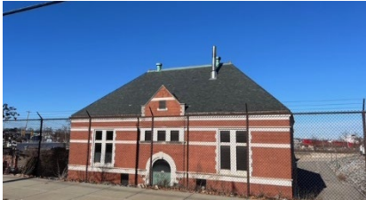
FPWWTF Ernest Street Pump
