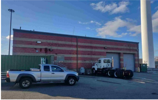
Photo: Sludge Dewatering and Handling Facility
