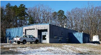
Lincoln Septage Receiving Station
