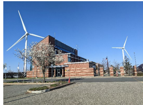
Field's Point Administration Building
