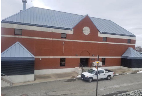
Photo: Ernest Street Pump Station
