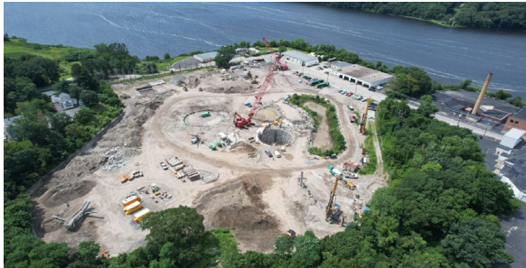
Photo: Pawtucket Tunnel Site
