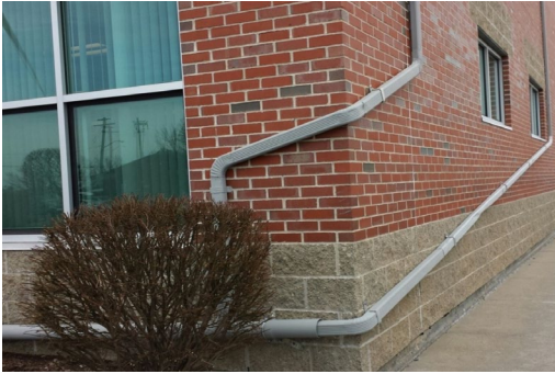
Photo: Downspouts at NBC's Corporate Office Building
