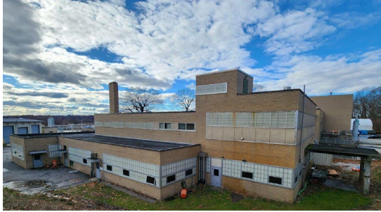
Photo: Bucklin Point Operations Building
