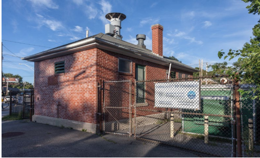
Photo: Reservoir Avenue Pump Station
