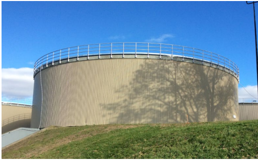
Photo: Bucklin Point Digester
