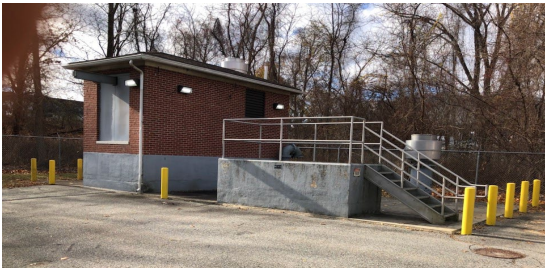
Photo: Saylesville Pump Station
