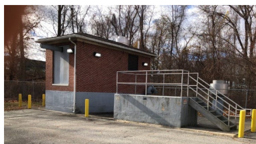
Saylesville Pump Station
