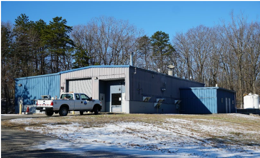
Photo: Lincoln Septage Receiving Station
