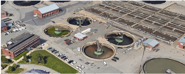
Photo: Wet Weather Clarifiers
