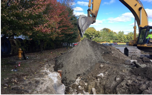
Photo: Construction on the Moshassuck Valley Interceptor
