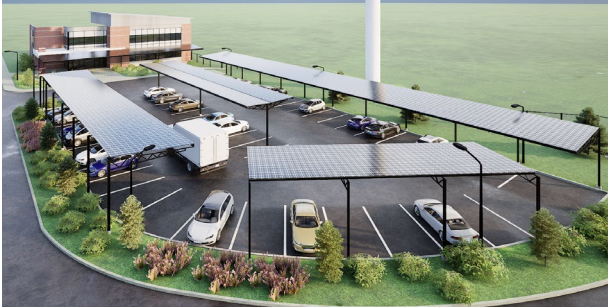
Photo: Solar Carport
