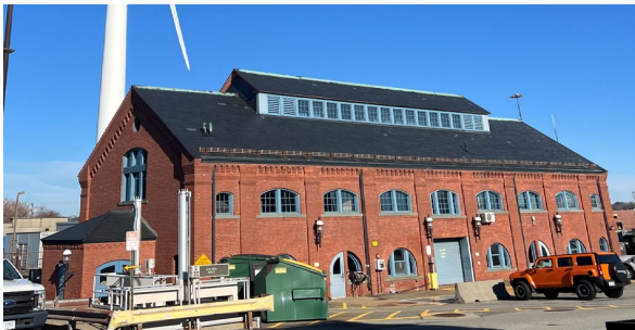
Photo: Existing FPWWTF Maintenance Building
