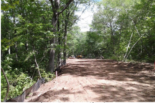
Photo: Easement Clearing
