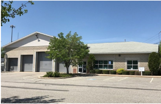
Photo: Interceptor Maintenance Building
